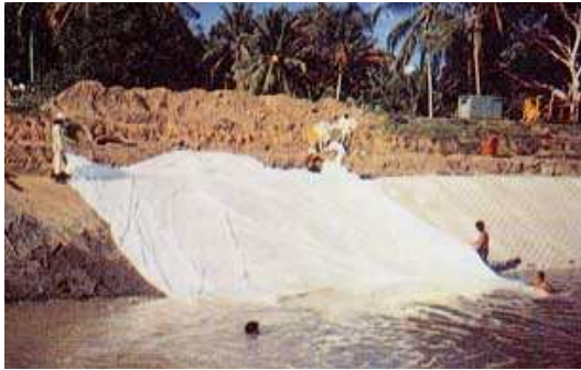
Figure 7: Laying a grouted mattress
