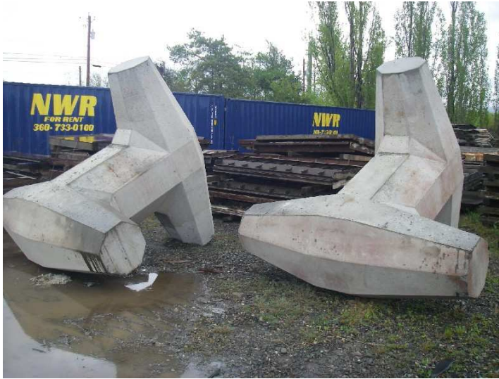
Figure 8: Showing concrete ‘dolos’
