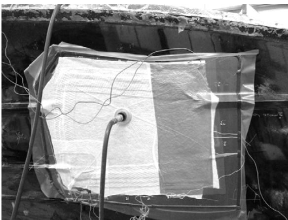
Figure 7.15: Fore repair joint prior to be insulated
