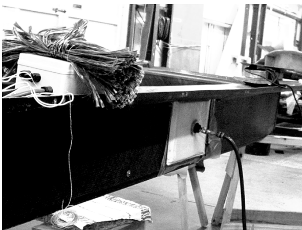
Figure 3.1: Flat panel repair on a simple geometry TPC boat (BAE Systems, Figure 2.2)
