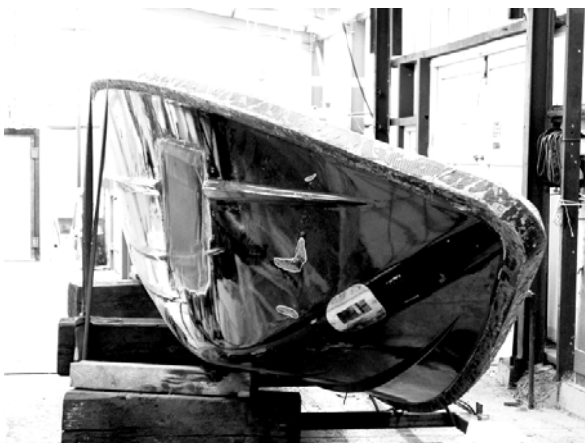
Figure 7.21: Fore view of the repaired hull
