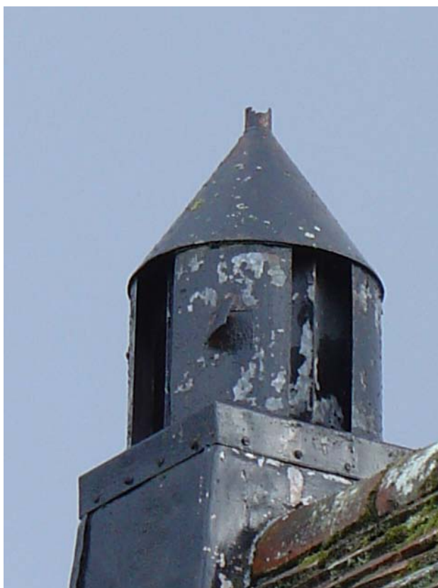
Figure 6-17 The chimney at School A
