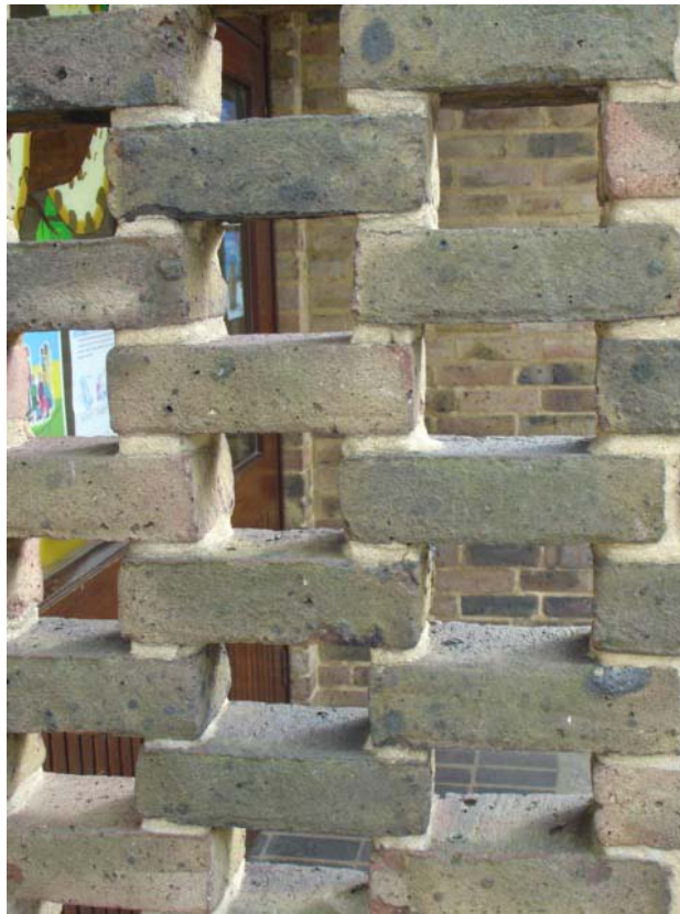
Figure 6-20 The playground wall at School S
