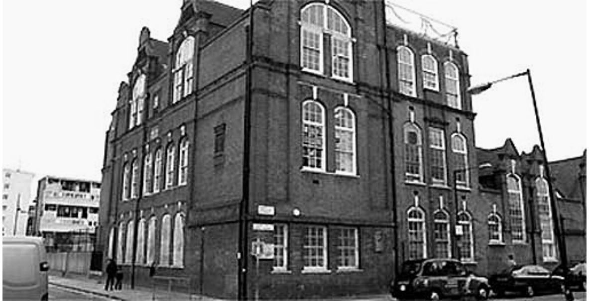
Figure 2-1 Bonner Street primary school, Tower Hamlets, London. Photograph: Graham Turner. Source: Weaver (2006)
