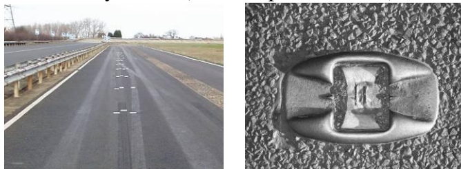
Expansion Joints (vehicle speed 16 km/h)
