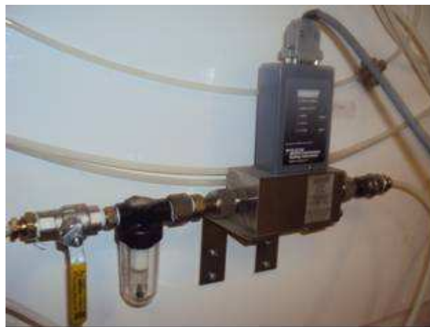
Figure 6-21: Thermal mass flowmeter
