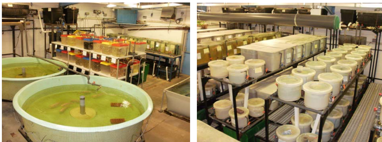
Figure 2.1 Water Recirculatory System in Tropical Aquarium Facilities, with spawning circular tanks and glass aquaria (L) and circular and rectangular fibreglass tanks (R).
