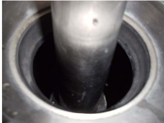
Figure 4: Product residues on filling pipe
