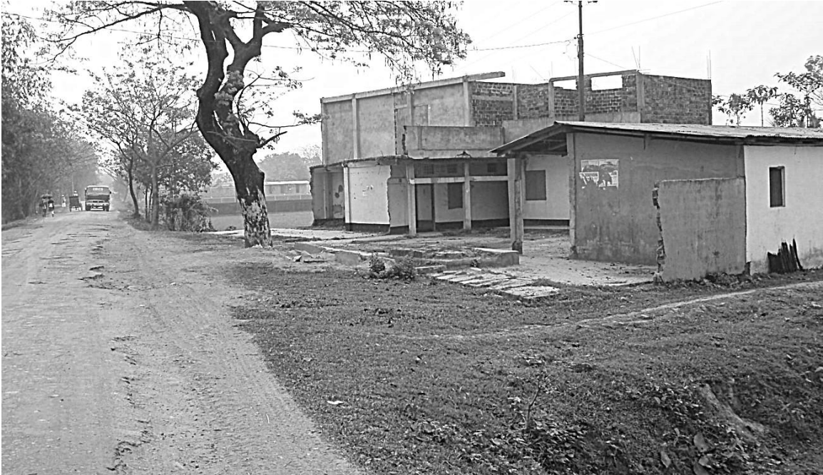
Plate 1: A demolished Bishwanath madrassa during the emergency.
