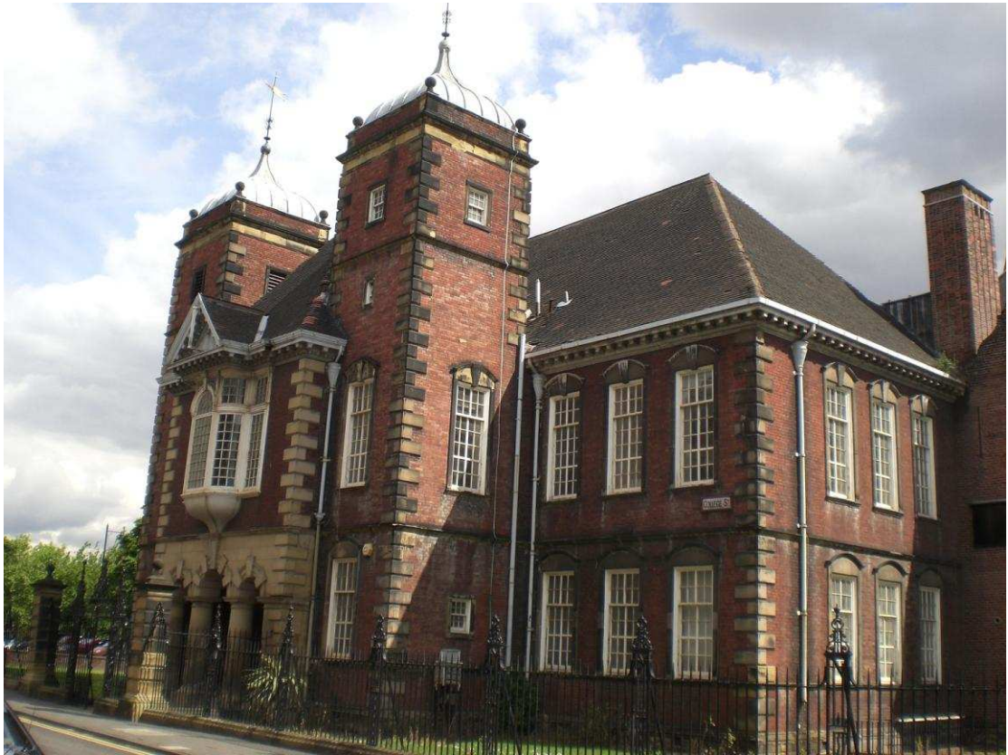
Figure 8 Dame Allan School, College Street, designed by R.J. Johnson, 1882. (Author's photograph).
