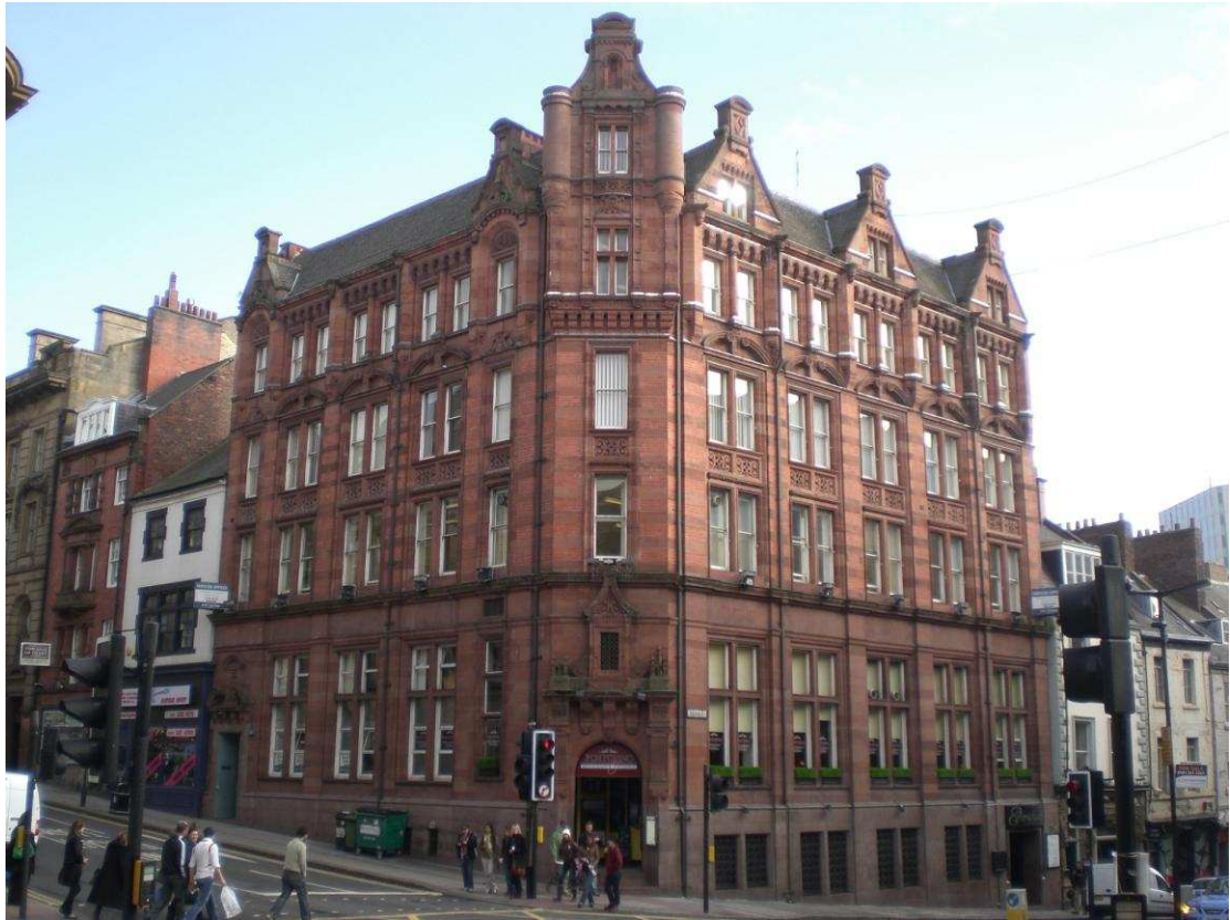
Figure 102 Prudential Assurance Company offices, designed by Alfred Waterhouse, 1891. (Author's photograph).
