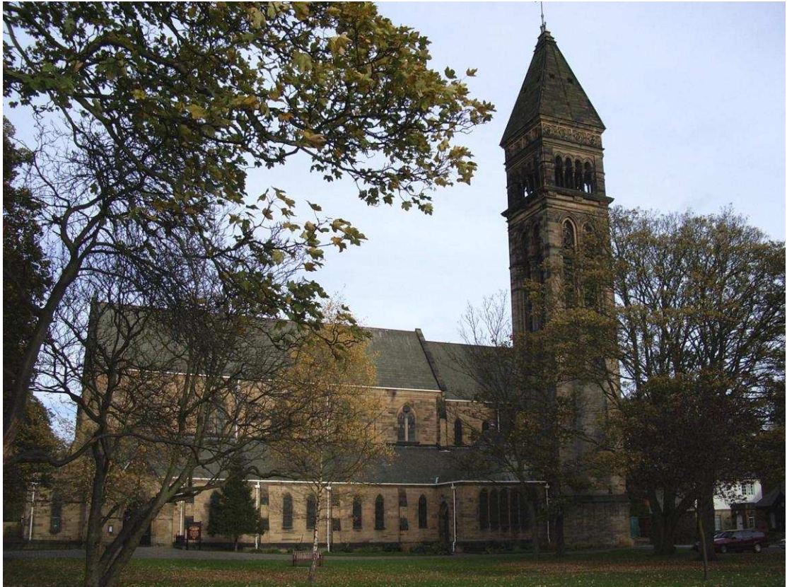
Figure 78 St. George's Church, Jesmond, designed by T.R. Spence, 1887-9. (Author's photograph).
