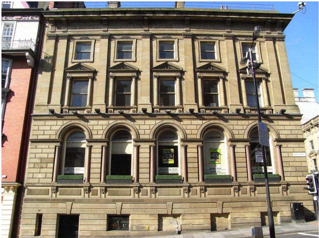
Figure 85 National Provincial Bank, designed by John Gibson, 1870-2. (Author's photograph).
