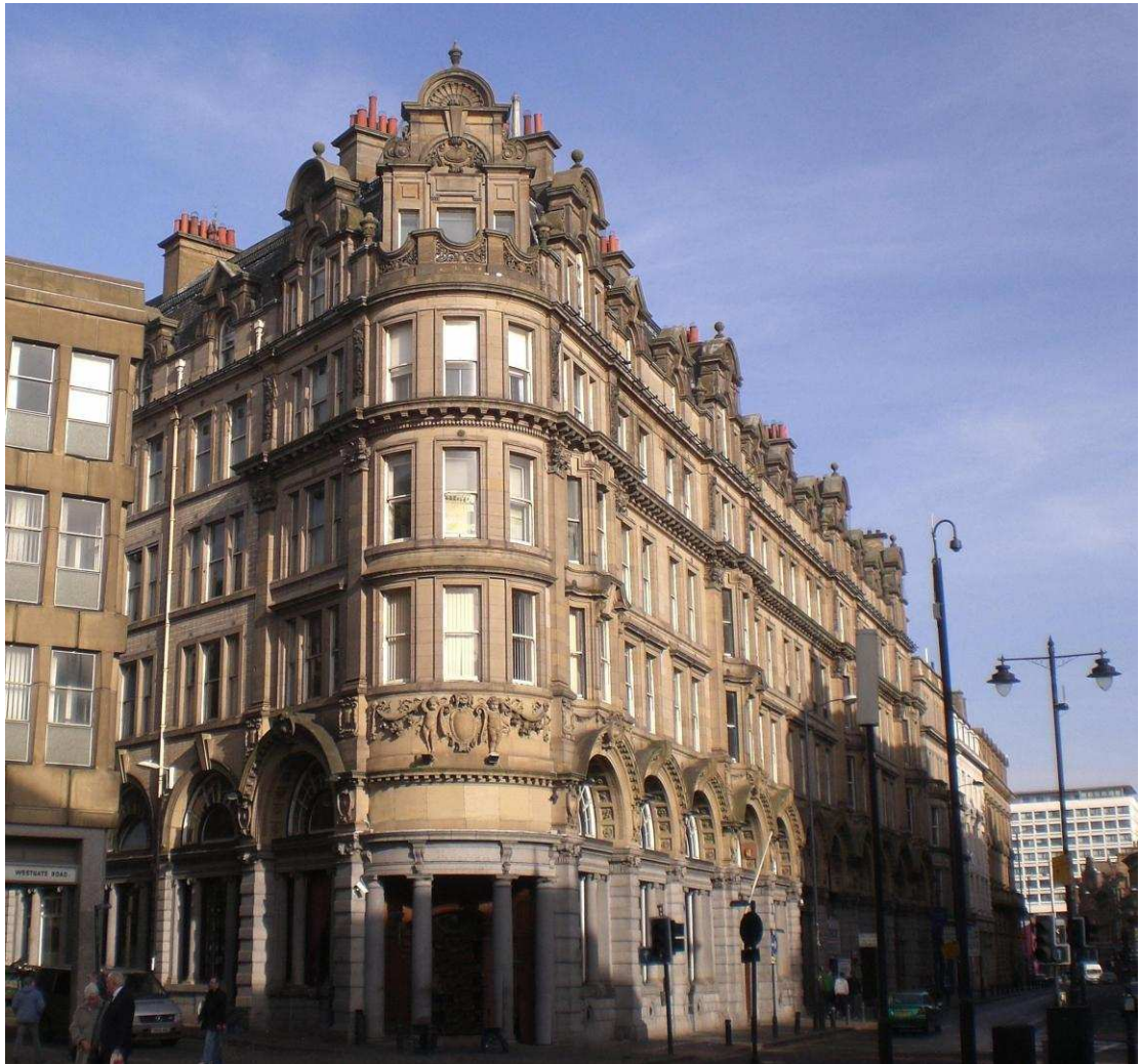
Figure 94 Collingwood Buildings, designed by Oliver and Leeson, 1897-9. (Author's photograph).
