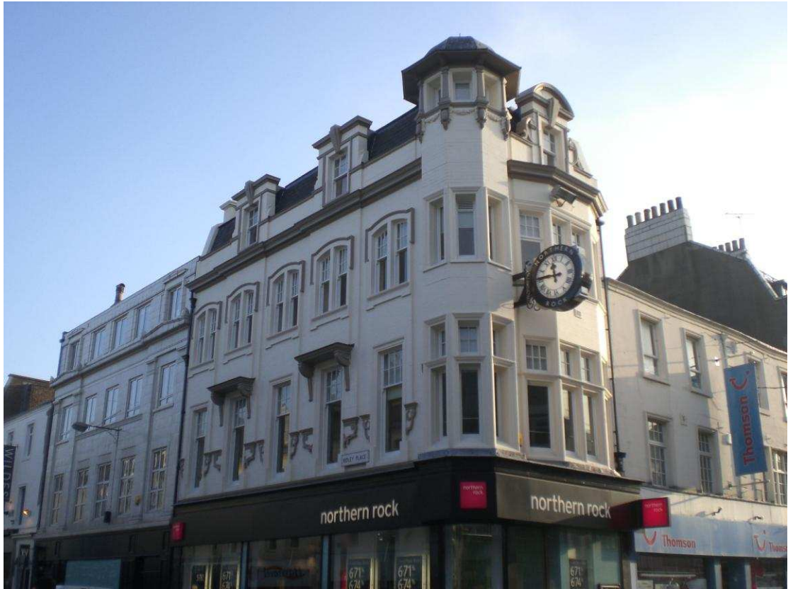
Figure 25 No. 132-134 Northumberland Street. (Author's photograph).
