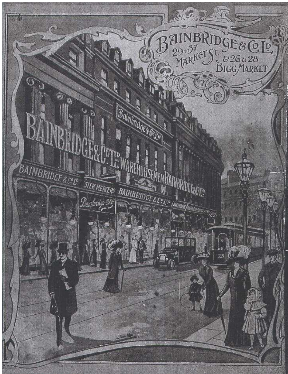
Figure 147 Bainbridge's arcade windows in 1912. (Bainbridge & Co. [1912] 'Clothing and Cap Making').
