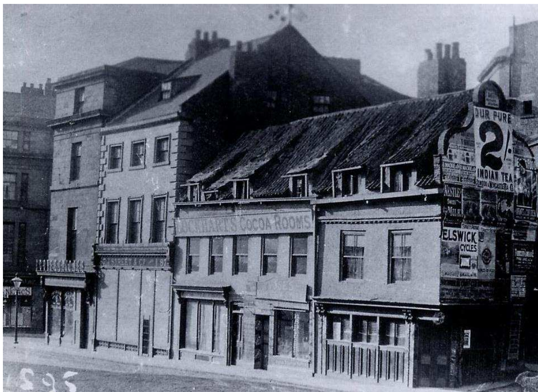
Figure 140 Lockhart, Smith and Co., original premises on Westgate Road. The plain Classical building on the corner was acquired by Northern Goldsmiths and remodelled in exuberant Baroque style. Hoardings on the side of the adjacent building testify to the growing importance of advertising media. (Jack Philips Photograph Collection).
