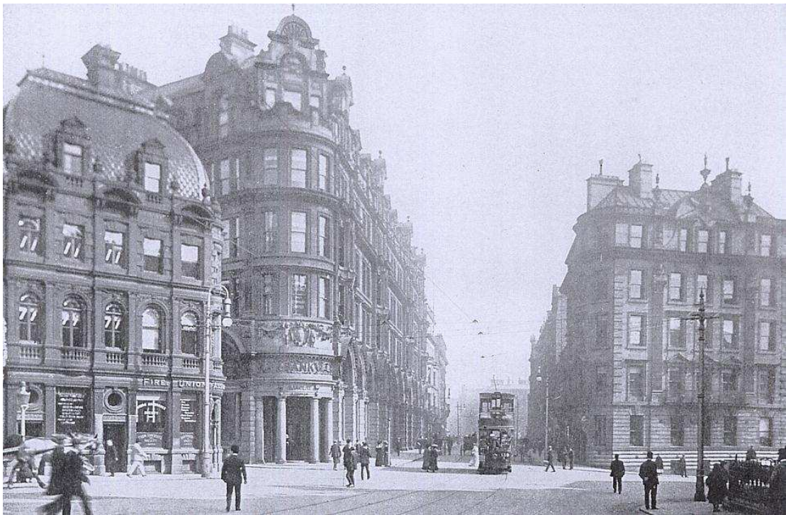
Figure 97 The western entrance to Collingwood Street, c.1912. The Collingwood Buildings and the Sun Insurance Company's offices frame the vista. (Mawson, Swan and Morgan [c.1912] Fine Art Photographic Views of Newcastle, Gateshead, Whitley Bay and District . Newcastle: Mawson, Swan and Morgan Ltd). This photograph was reused as a postcard.
