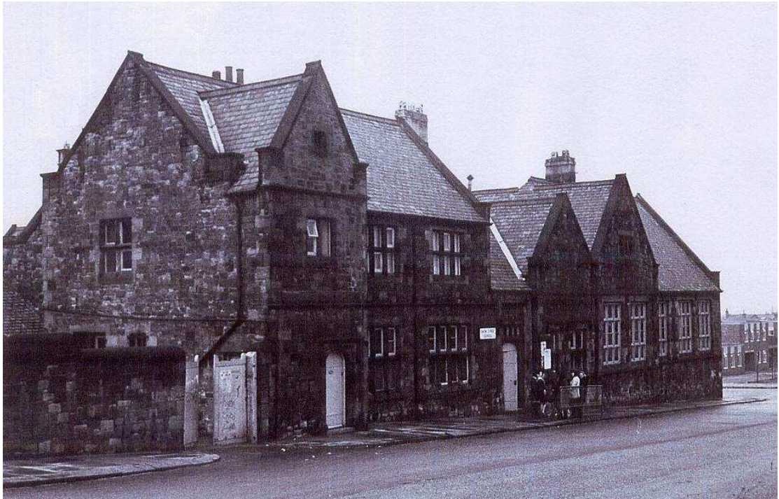
Figure 155 Arthur's Hill Board School, Snow Street, designed by R.J. Johnson, 1873-5. (Newcastle City Library).
