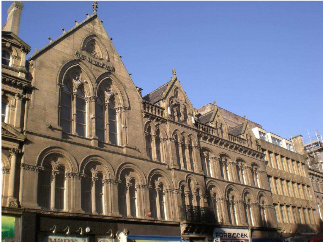
Figure 119 Chaucer Buildings, Nos. 53-61 Grainger Street West, by Gibson Kyle, c.1869. (Author's photograph).
