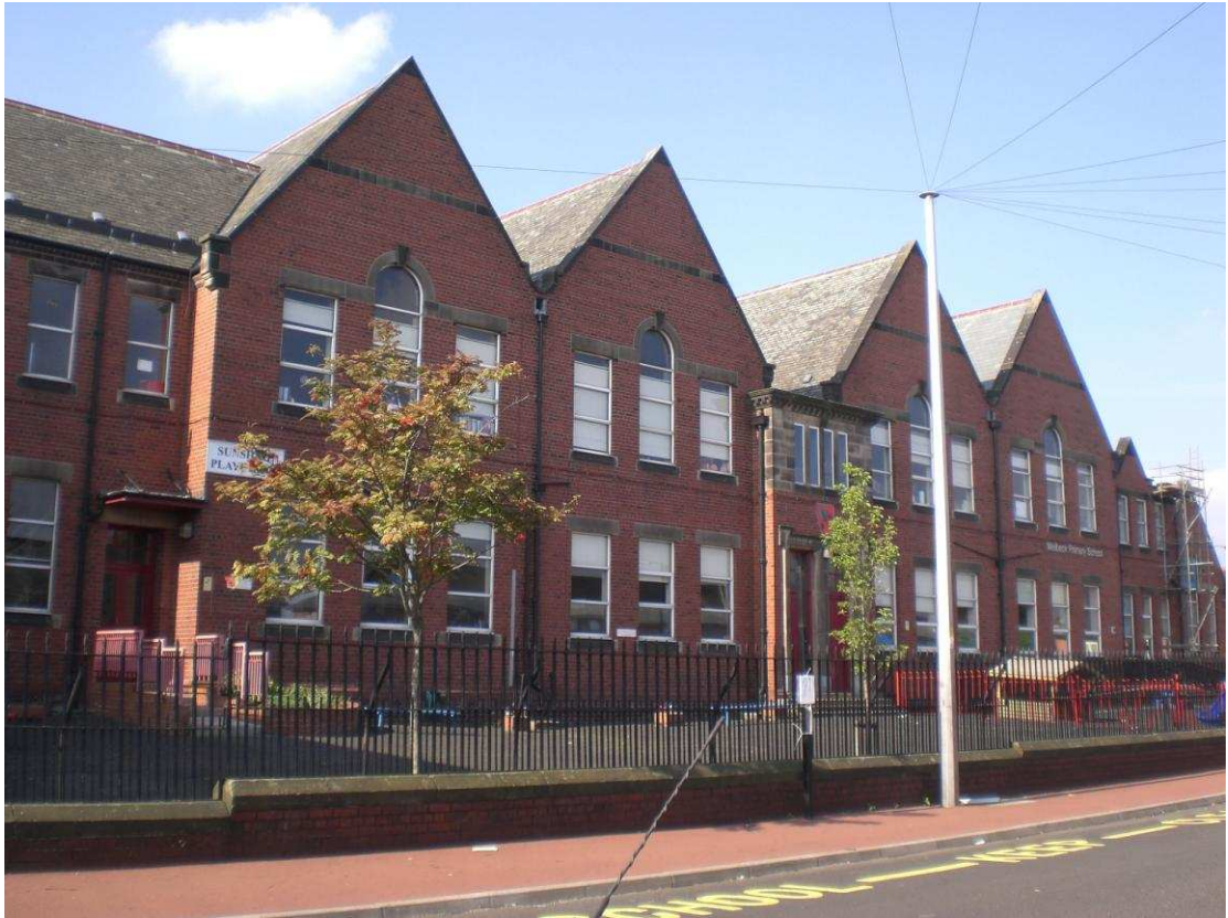
Figure 164 Welbeck Road School, designed by W.H. Knowles, executed 1905-6. (Author's photograph).
