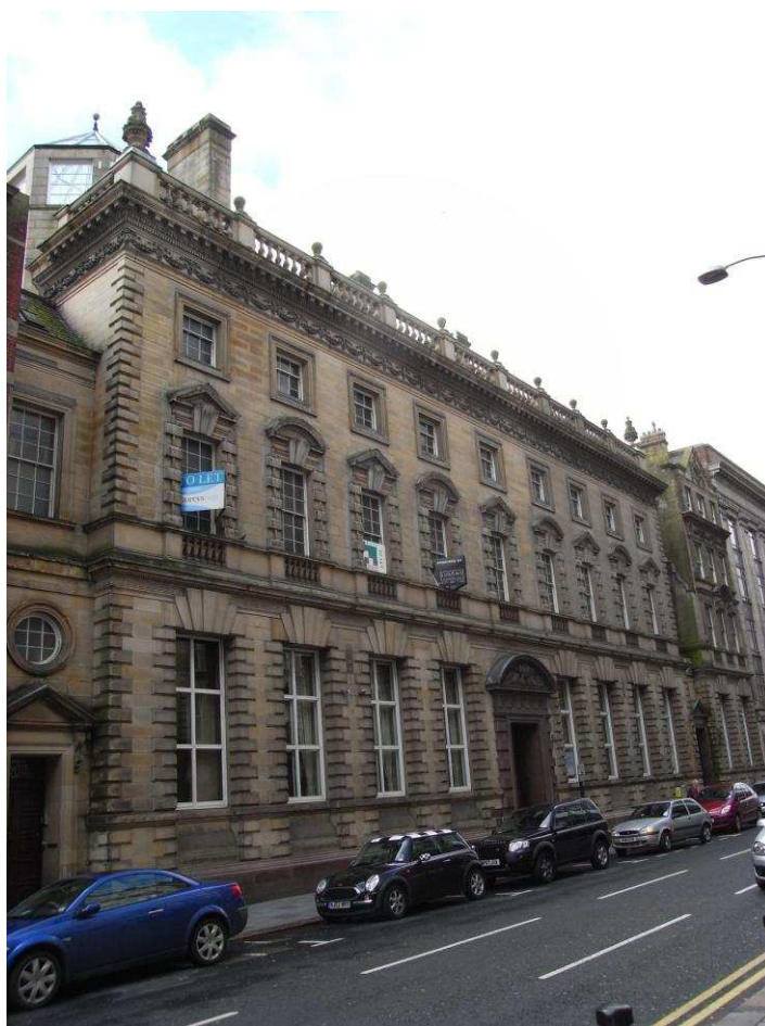
Figure 88 Hodgkin, Barnett, Spence, Pease and Co.'s Bank, Collingwood Street, designed by R.J. Johnson, 1888-92. (Author's photograph).
