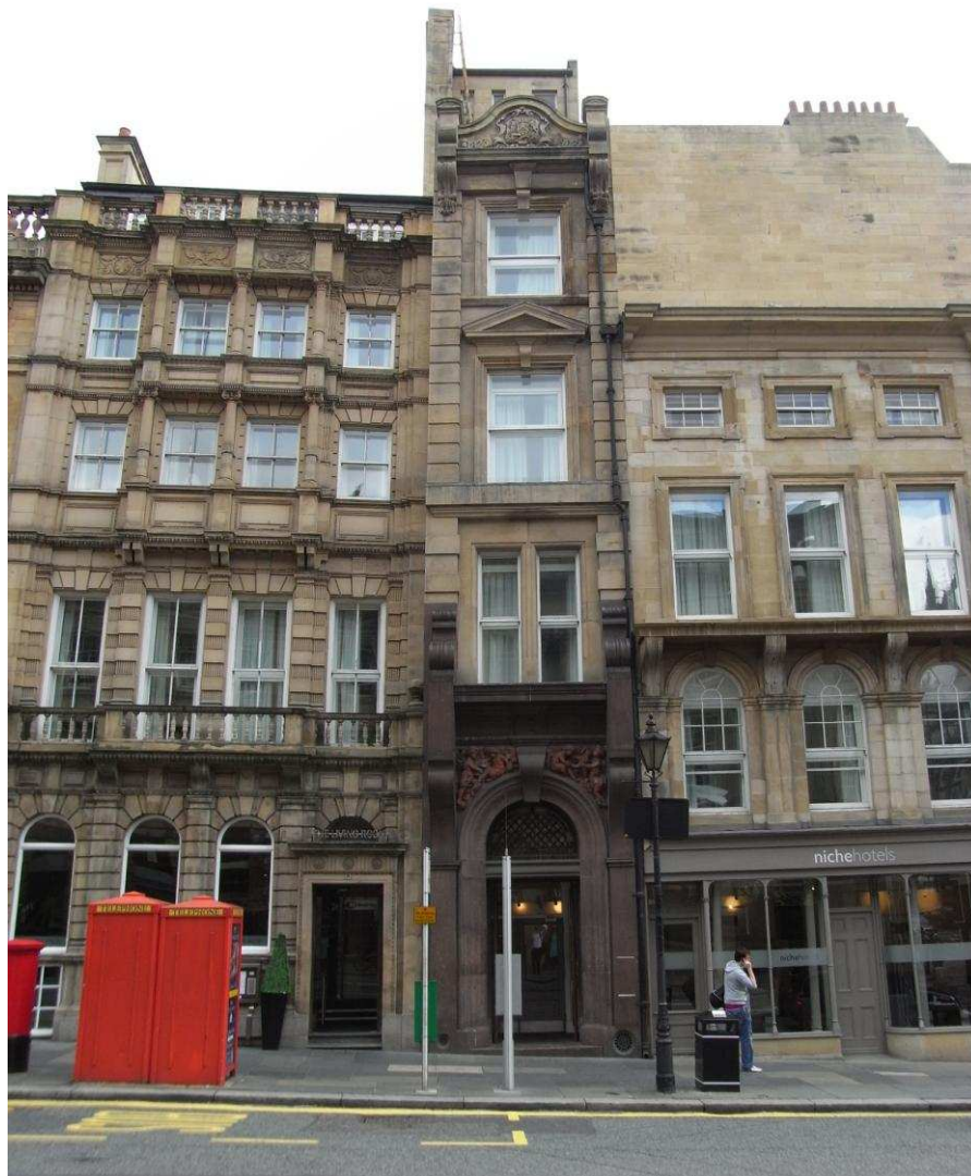
Figure 105 Edinburgh Life Assurance Company offices, No. 10 Grey Street, designed by Fred T. Walker, 1906-8. (Author's photograph).
