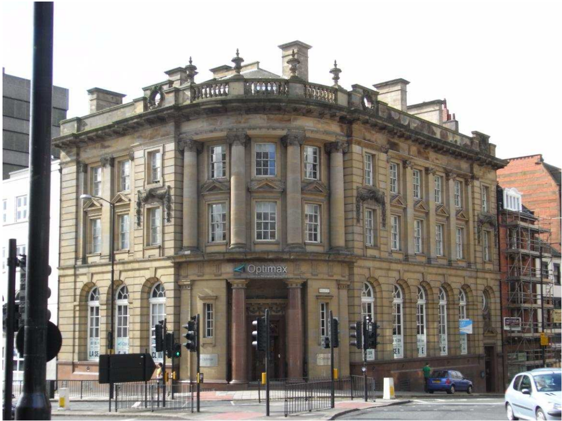
Figure 106 Alliance Assurance Company offices, Nos. 2 and 4 Mosley Street, designed by Newcombe and Newcombe. (Author's photograph).
