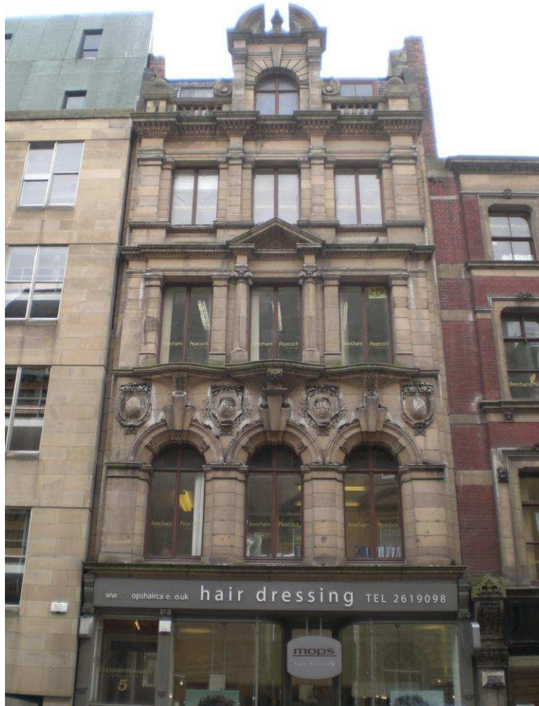
Figure 98 J.C. Eno's premises, No. 5 Collingwood Street, designed by J.W. Taylor, 1900. (Author's photograph).
