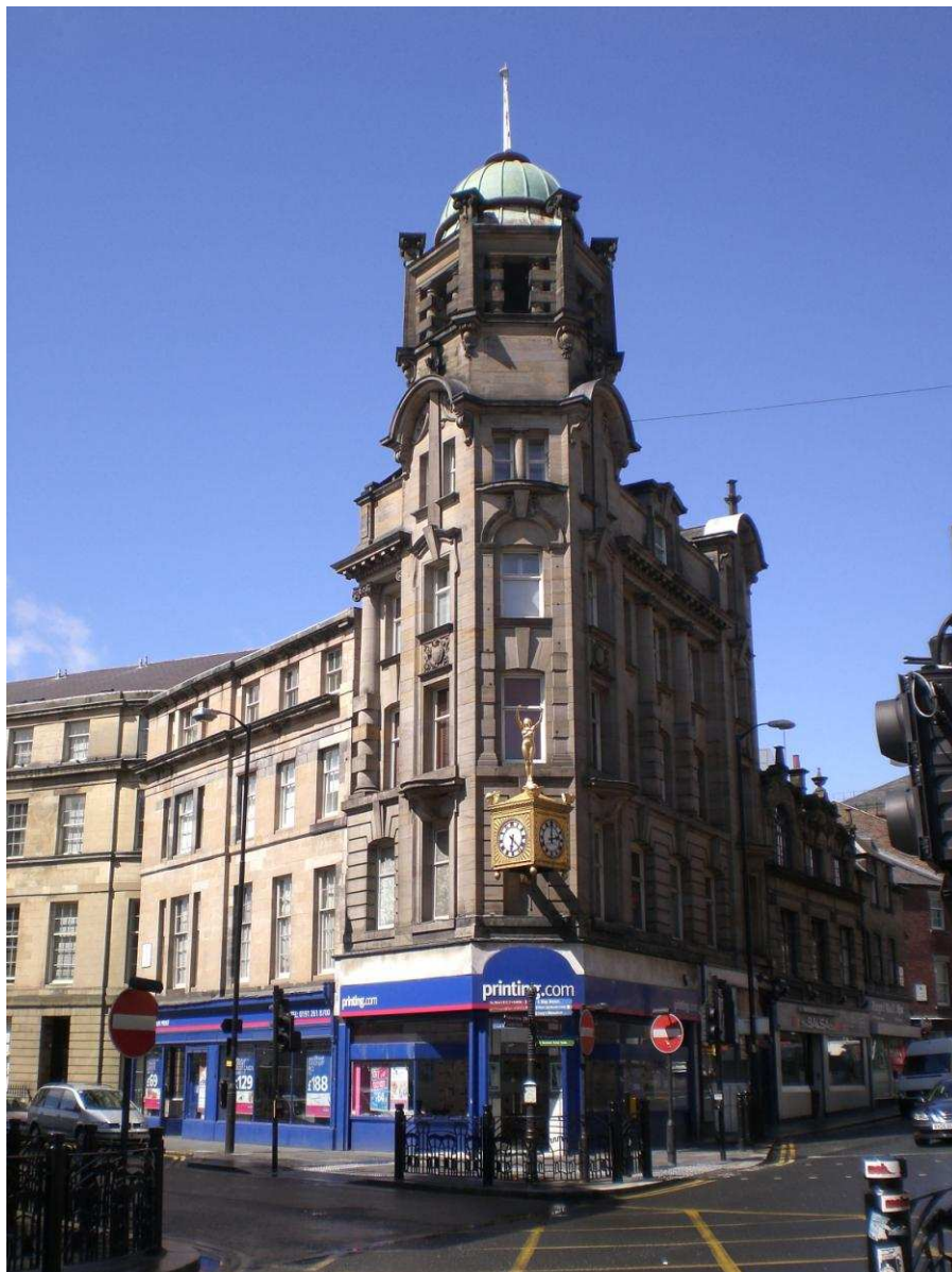
Figure 142 Northern Goldsmiths' premises, Westgate Road, designed by Cackett and Burns Dick, c.1910. (Author's photograph).
