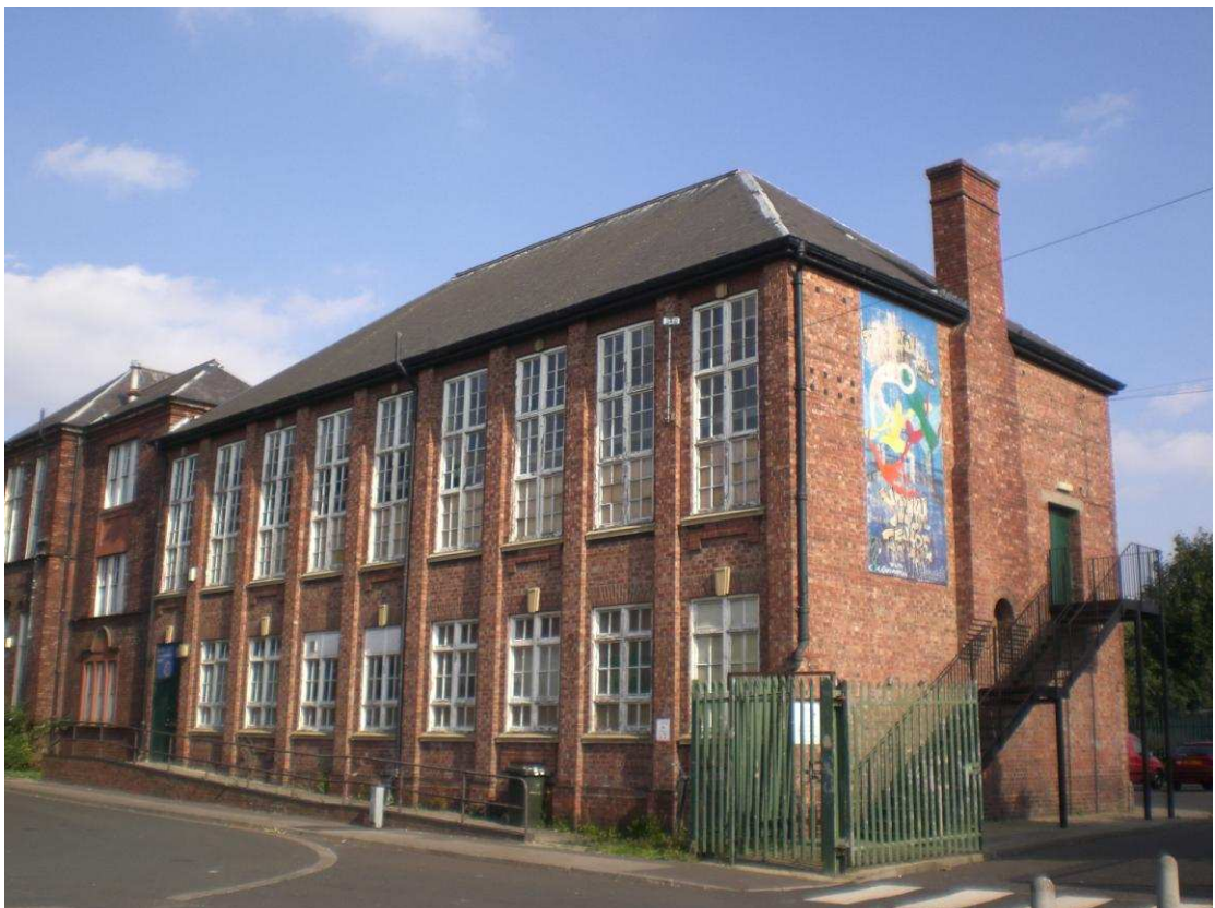
Figure 6 Raby Street Board School, Byker, designed by W. L. Newcombe, 1895-7. (Author's photograph).
