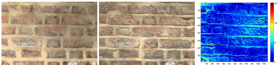
(a) Albedo maps: From left to right, captured, histogram matched, difference image
