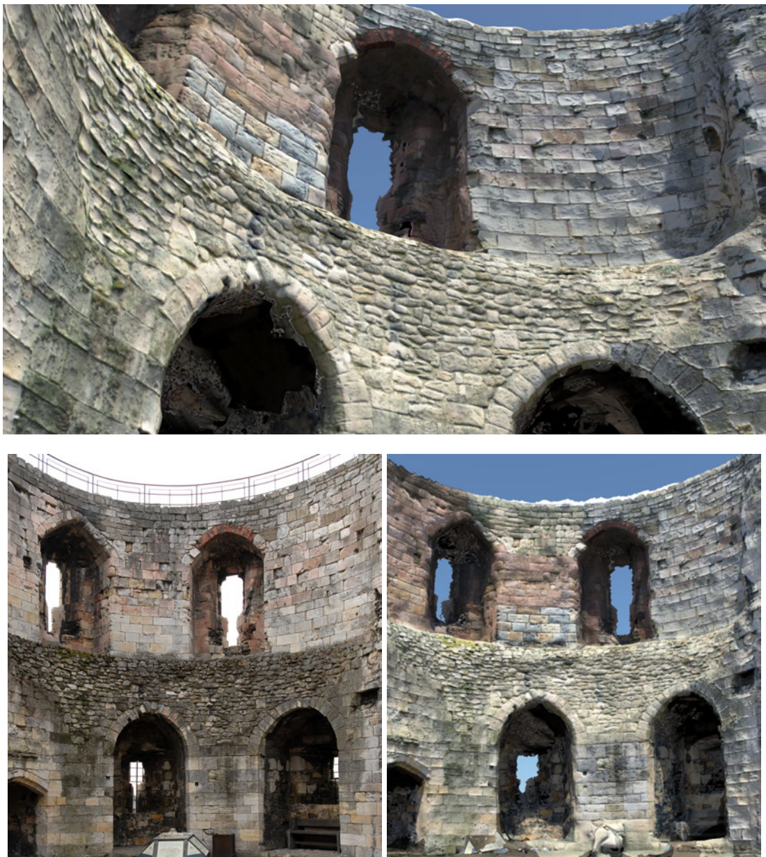
Figure 6.15: Interior façade of the Clifford's Tower Model (top and bottom-right), compared with a photograph of the real façade (bottom-left).
