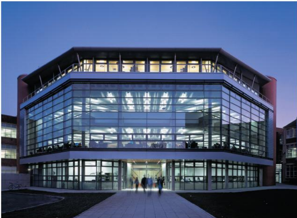
Figure 8.1d Approach view of MI Building:
