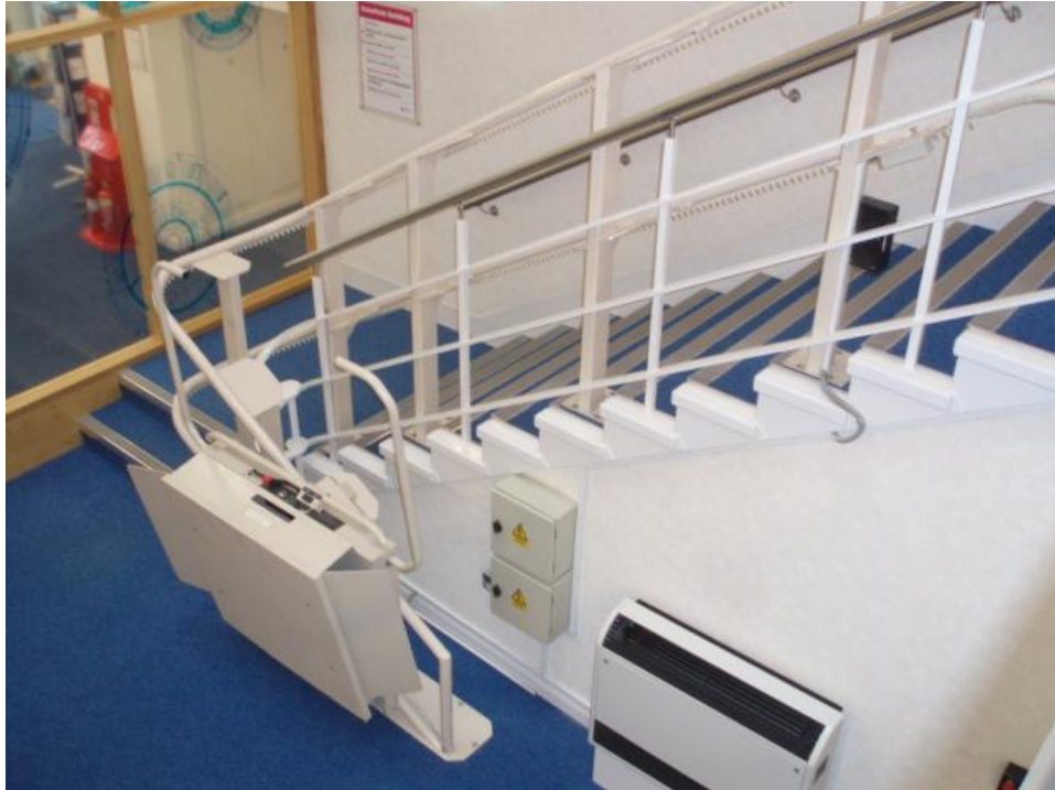
Figure 8.3c Stair lift to upper floor for disabled users Loughborough University Sigma Mathematics Support Centre: source Adejumo F.T ELSD photo gallery, 2007
