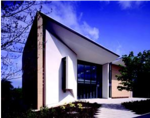
Fig 4.4a University of Reading's ISMA banking research building an example of a Cost model: 21st-century university building:
