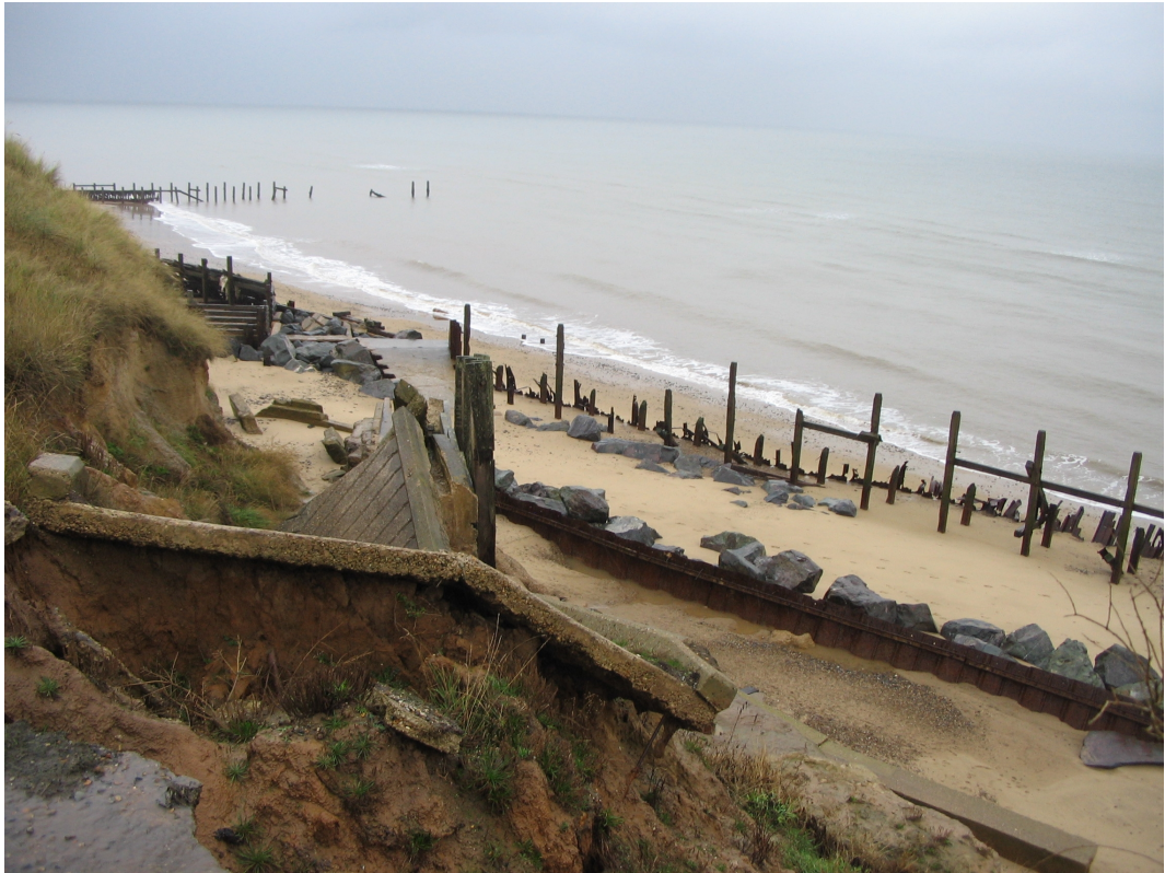
Figure 8.2: Coastal erosion at Happisburgh, Norfolk
