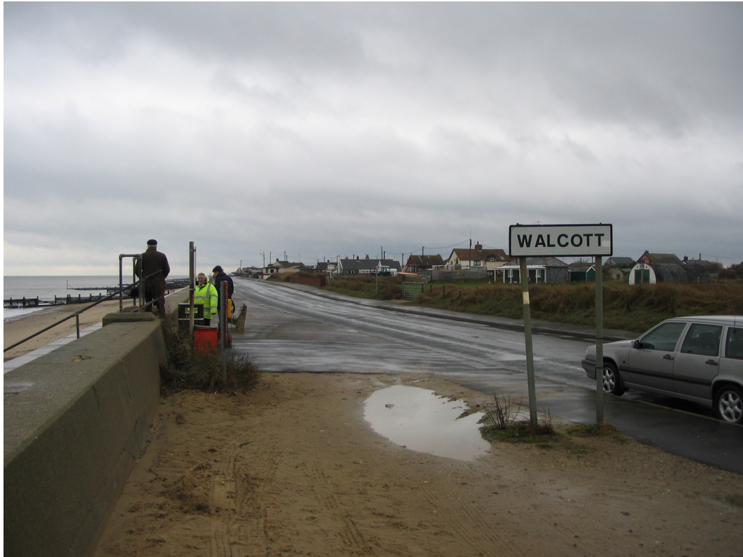
Figure 8.8: Looking southeast along seawall, showing low-lying coastal road and Walcott village
