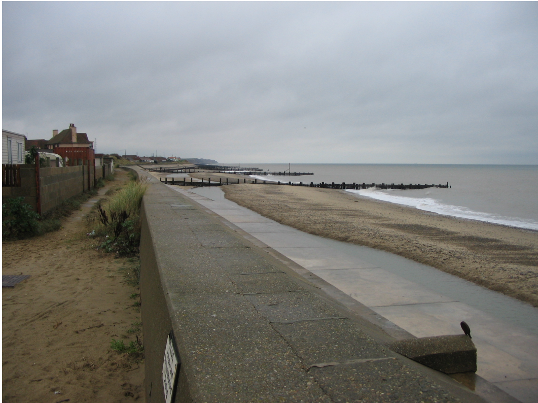
Figure 8.7: Looking northwest along seawall, showing sand/flint beach and groynes
