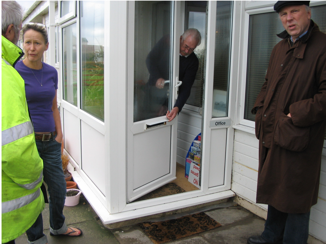
Figure 8.4: Walcott Caravan Park office, showing maximum flood levels on 9th November 2007
