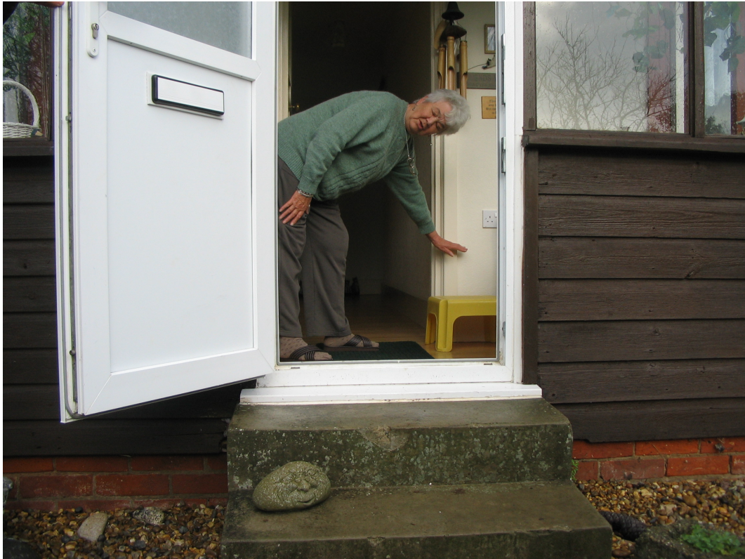
Figure 8.6: Reported maximum flood level, from a location near the Hundred Drain
