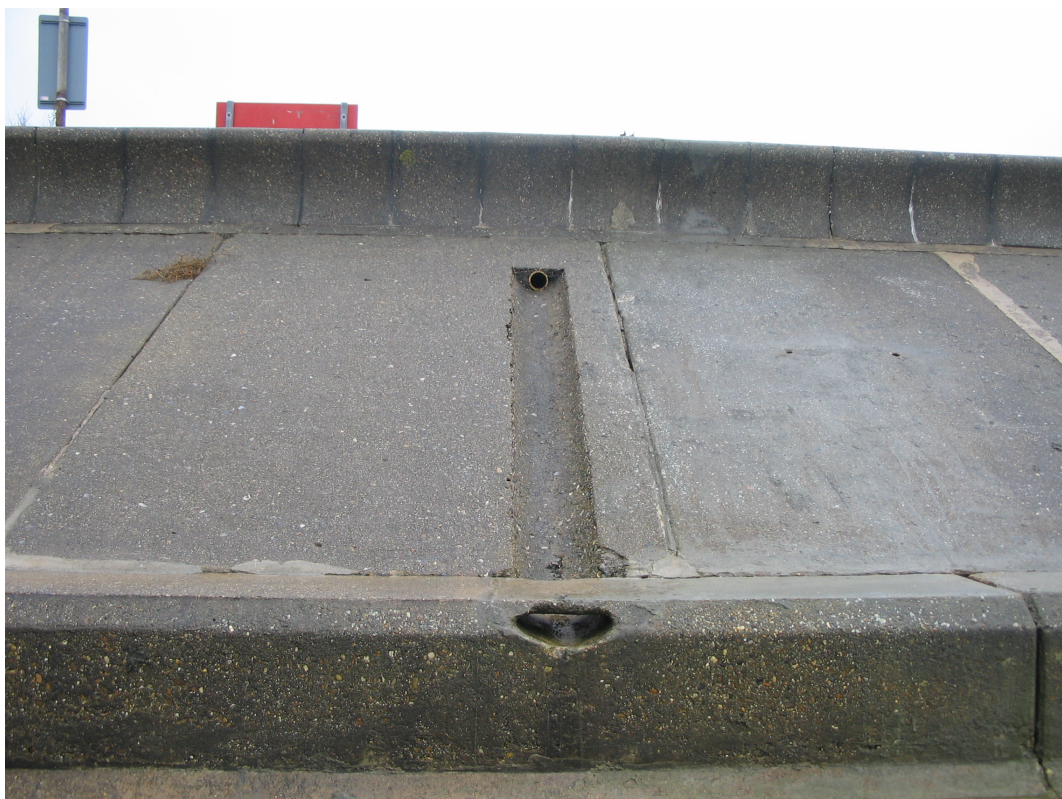
Figure 8.9: Looking at seawall from beach, showing road drain outfall
