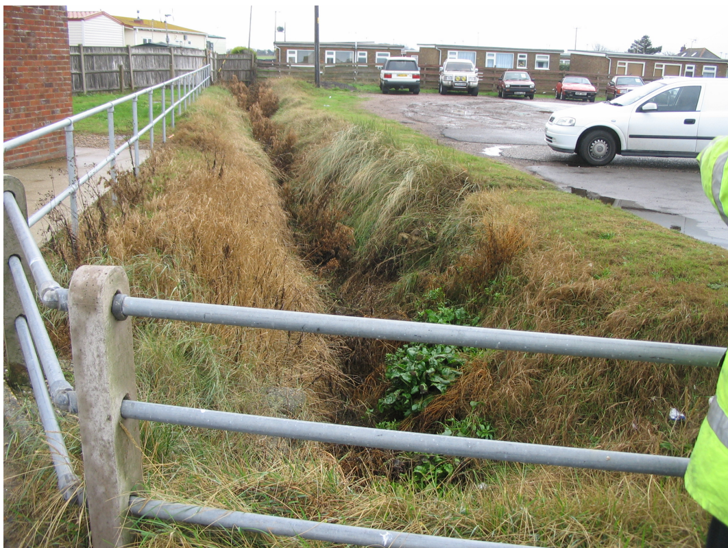
Figure 8.5: Hundred Drain, near Walcott seawall
