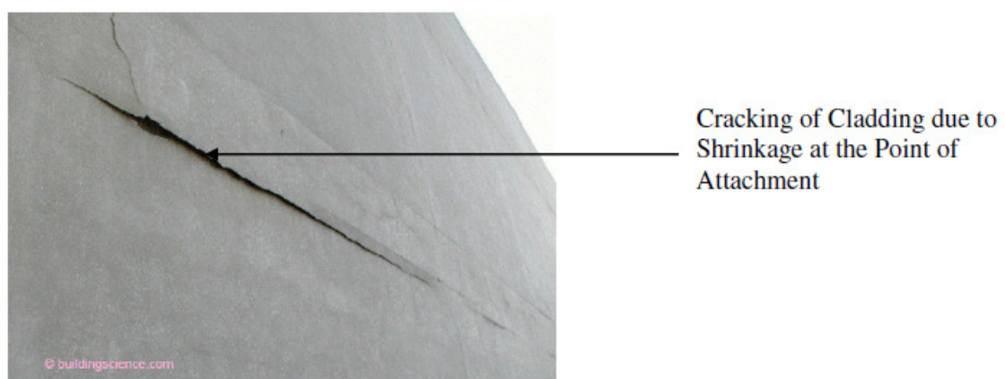
Figure 2.3. Frame shrinkage due to temperature variation [39]
