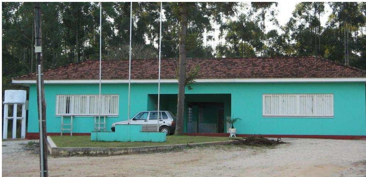
Figure 3.2.3.3d. “Fazenda Campininha”, Mogi Guaçu CU, main building (photo by the author, 2007)
