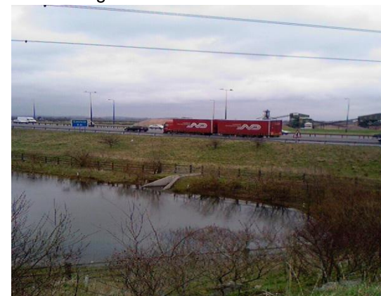
Photo 4.4 4 th sample point. The lagoon showing concrete outlet structure on far side of photograph. Sample point was taken 1/3 of the way around the perimeter of the lagoon.
