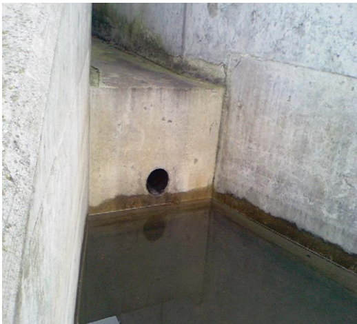
Photo 4.5 Outflow control structure
