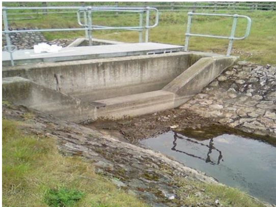
Photo 4.3 3 rd sample point. Outlet from the oil-separator showing the reverse side of the concrete underflow weir shown in Photo 4.2. No flow during dry conditions.
