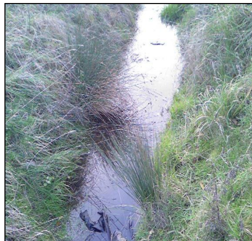
Photo 4.6 Ditch running alongside the M1
