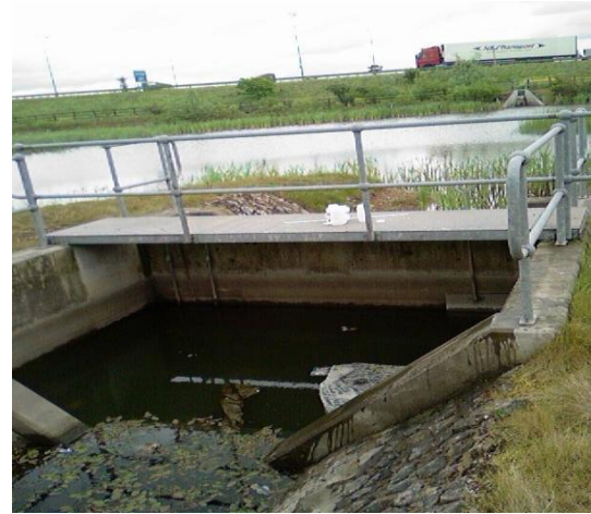
Photo 4.2 2 nd sample point. Inlet to the oil-separator showing underflow concrete weir. Lagoon and the M1 in background
