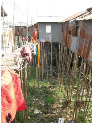
Figure 4-3: Pataton structure in Dhaka slums (bamboo, elevated structure 3-6 meters high over wasteland/water)
