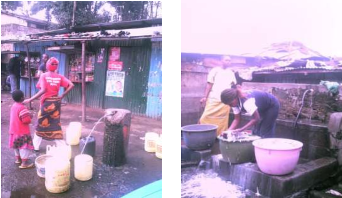
Figure 6-3: Standpipes in Pumwani after St. John's rehabilitated the water supply system
