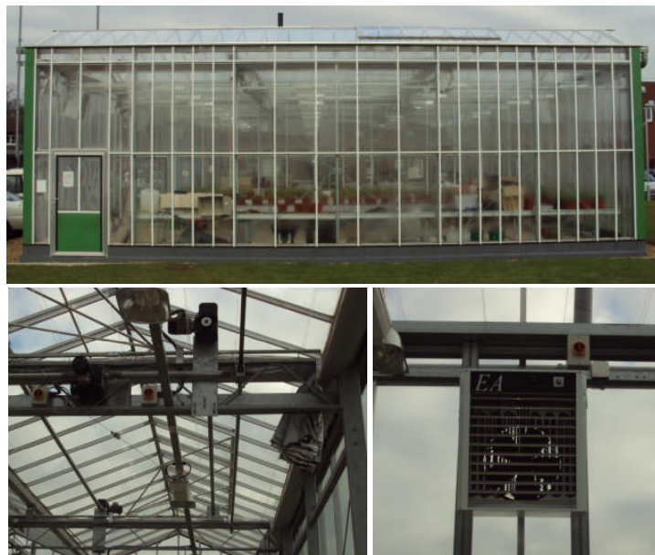
Figure A.6.1: Overview of the glasshouse facility at Cranfield University (top), close-up of the shade-cloth running on the horizontal frame along the roof (bottom-left) and close-up of a fan (bottom-right).
