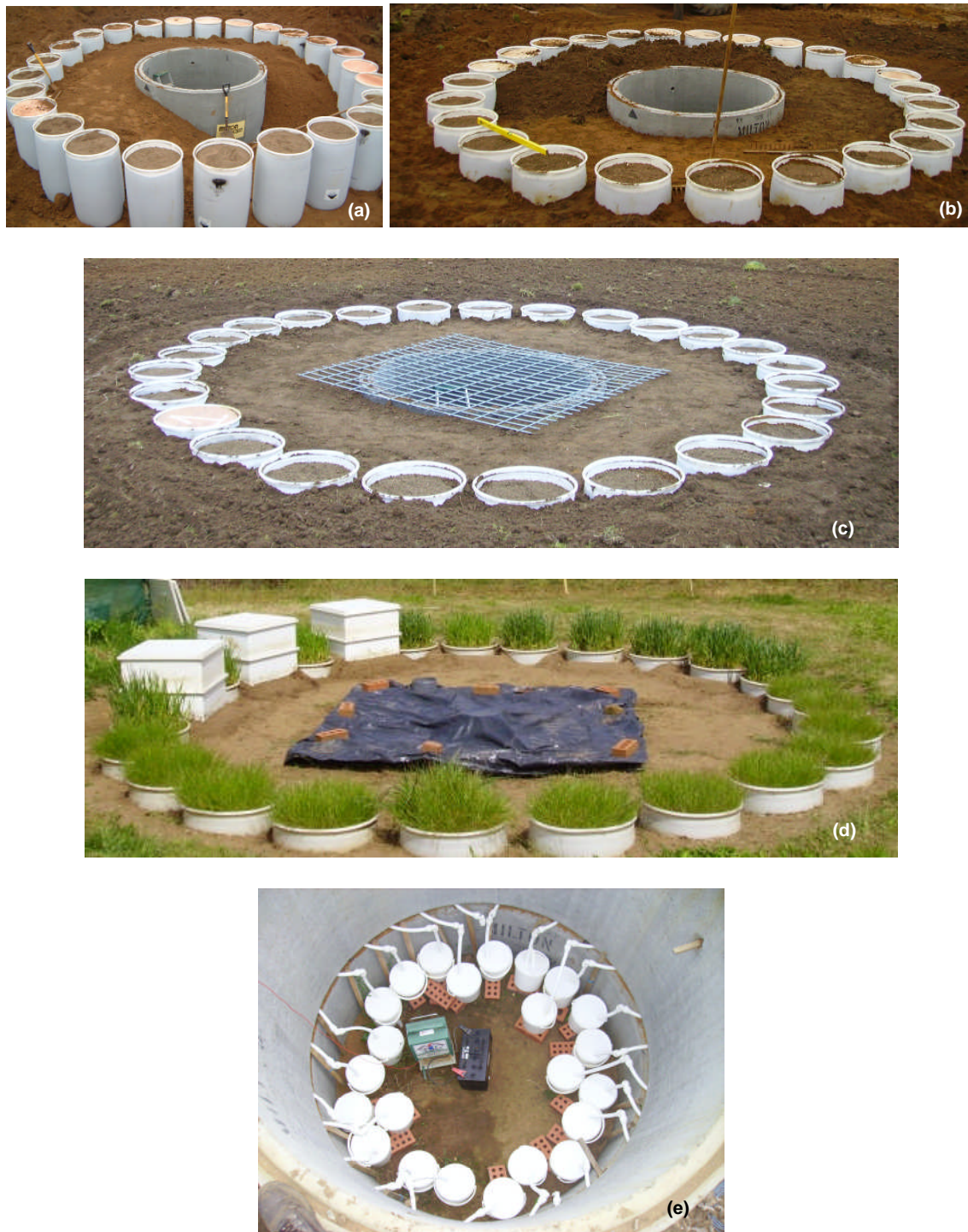
Figure A.1.2: Photographic record of lysimeters station at the College Farm; (a, b, c) construction (February 2008); (d) established crops and measurement of N_2O (May 2010); (e) view of the drainage and leachate collectors.
