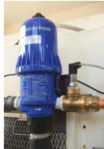
Figure 86 Dosatron body with pressure sensor to the right
