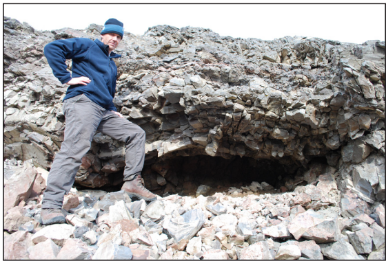
Fig. 4. F2. Cavities up to 1 m in width are present in the base of the unit.
