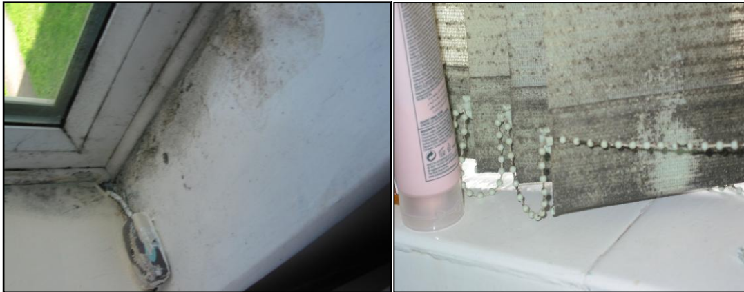
Plate 3.4 Fungal contamination on the bedroom window sill and bathroom blinds, Cranfield High Street
