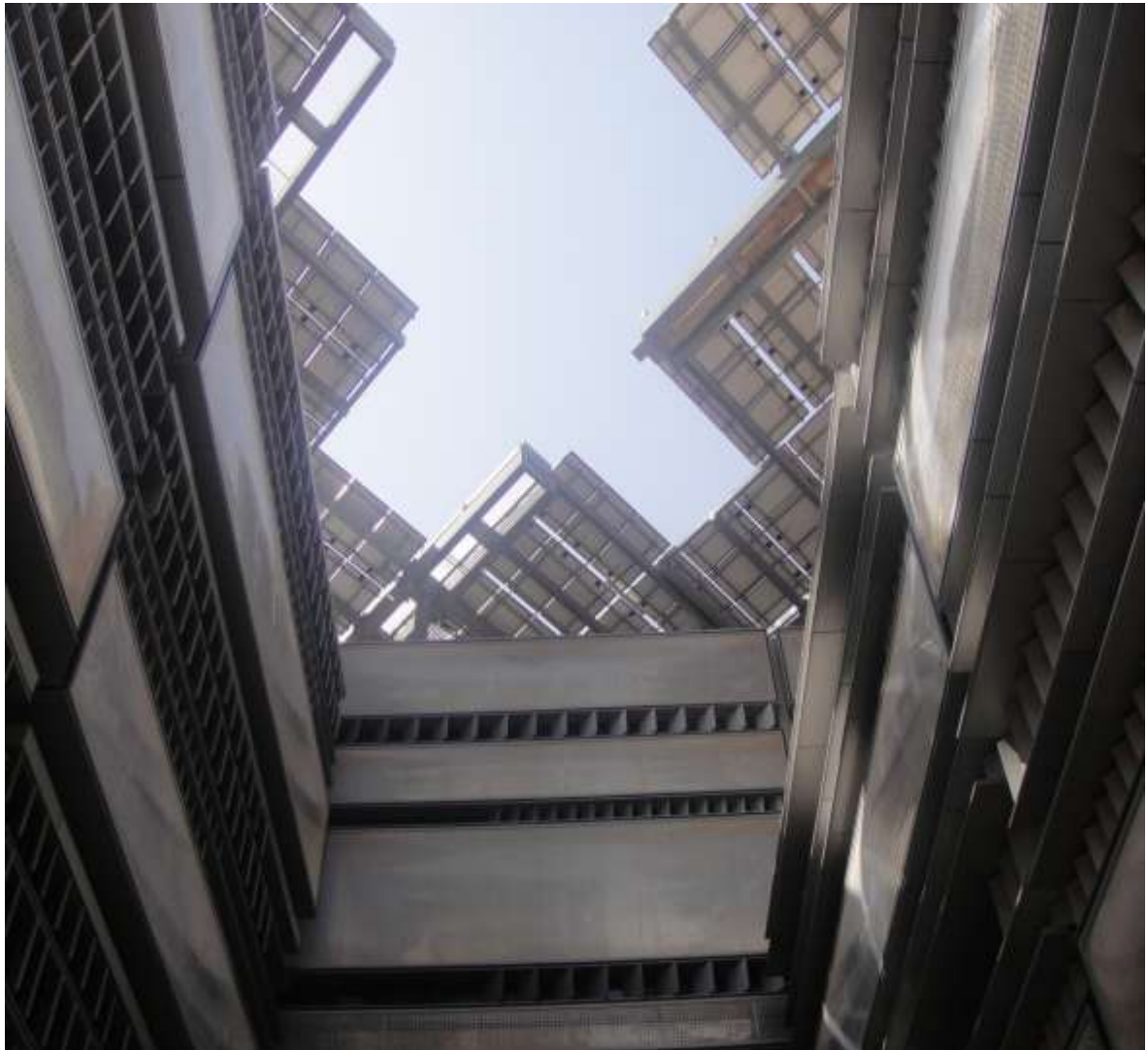
Figure 7.17: Shaded narrow outdoor corridors shaded with photovoltaic cells and surrounded by super-insulated walls, the Masdar Institute
