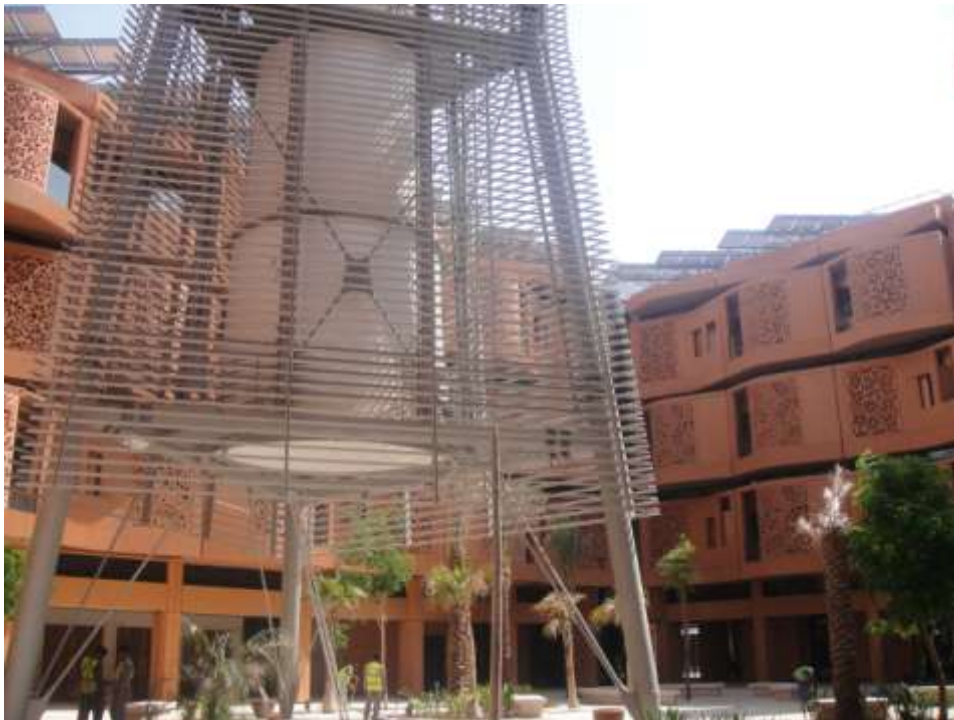
Figure7.3: Wind tower in the main courtyard of Masdar, designed to suck hot air upwards
