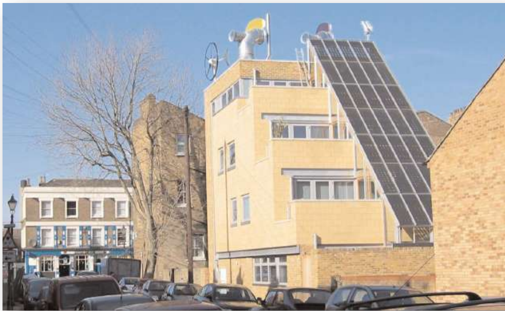
Figure 3.21: Bow Zed's PV laminate glazed sunspaces Source: ZED Factory, (2010)
