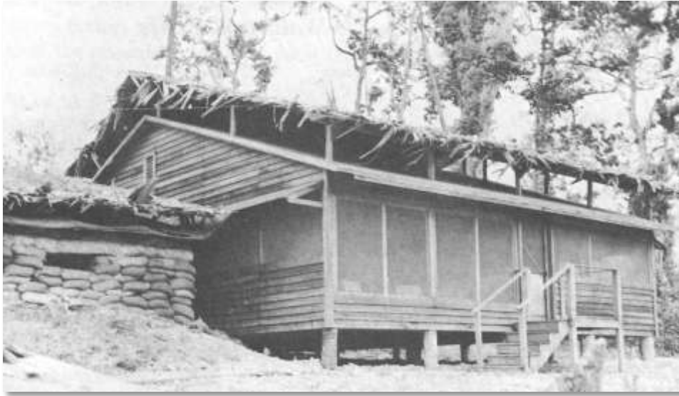
Figure 3.11: Air cooled roof in a hot humid climate, 1951 Source: Rogers, 1964, p.18
