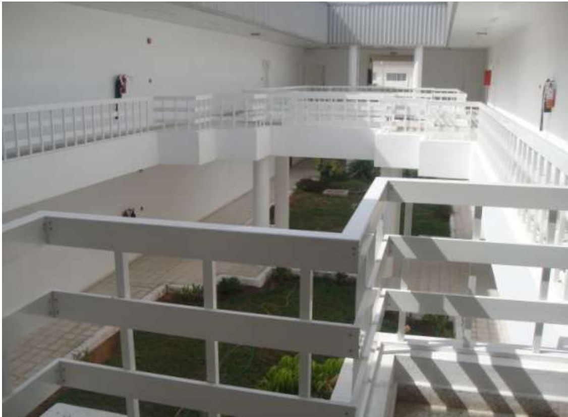
Figure7.12: Balconies, corridors and courtyard of the Educational Building
