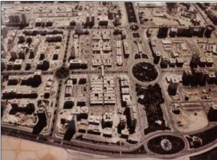
Figure 5.23: of the prevailing building style in Abu Dhabi during the sixties Source: Makhloof, 2006..
