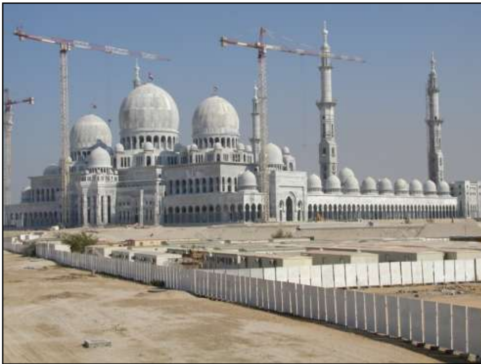
Figure 5.32: The Grand Mosque of Sheikh Zayed during construction
