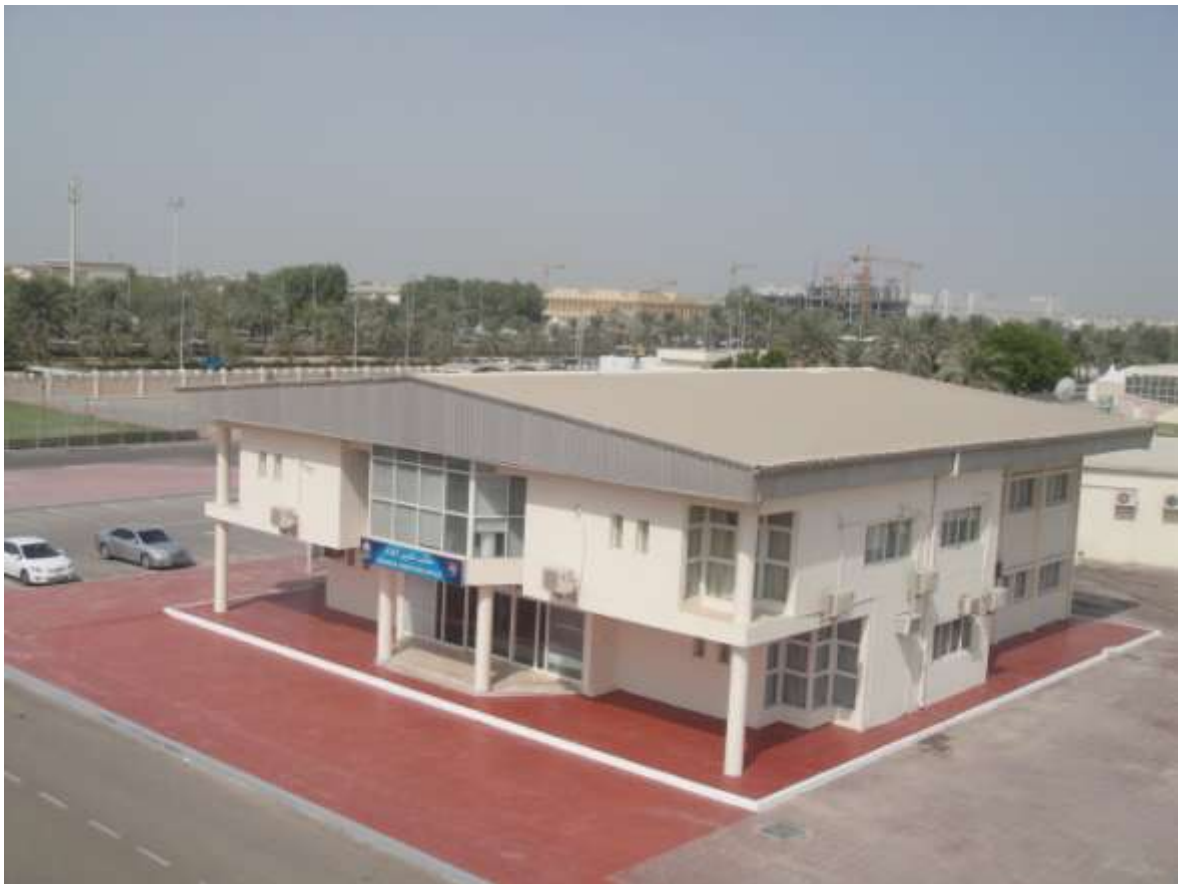
Figure 7.4: Police Academy Administrative building
