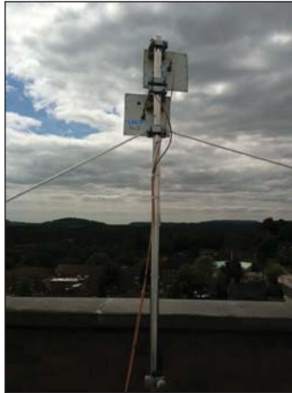
Figure 6.12: Photograph of the transmit antennas used in Bishops Court measurement.
