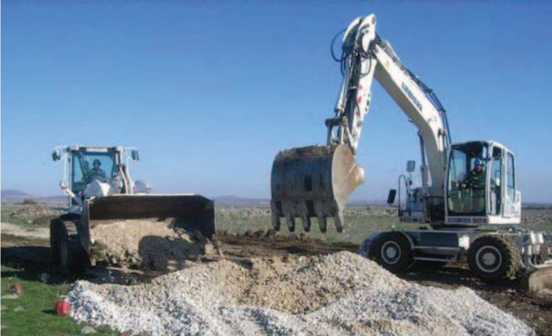
J-CON Road Repairs
