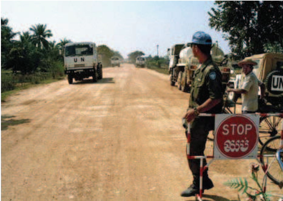
JSDF Road Repairs
