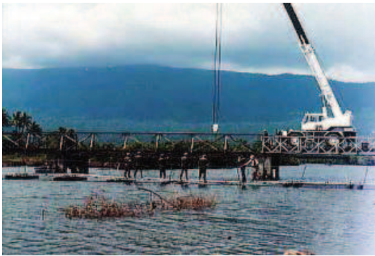
Repairing Route 3 Bridge
