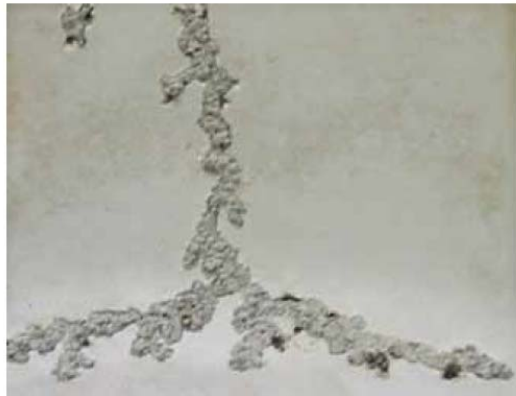
Figure 2.4: Degradation trace on polymeric insulator surface [54]
