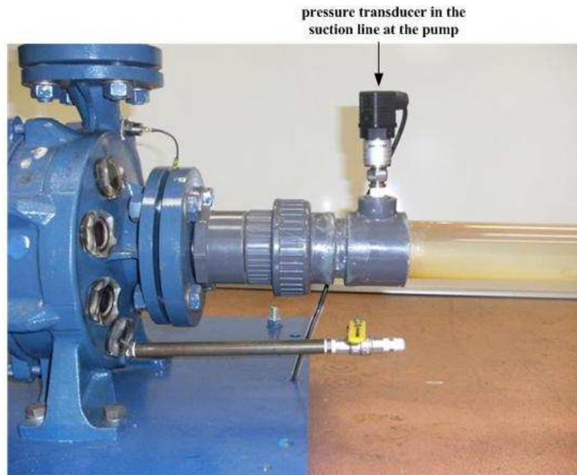
Figure 4-8 Pressure transducer in suction line at the pump inlet
