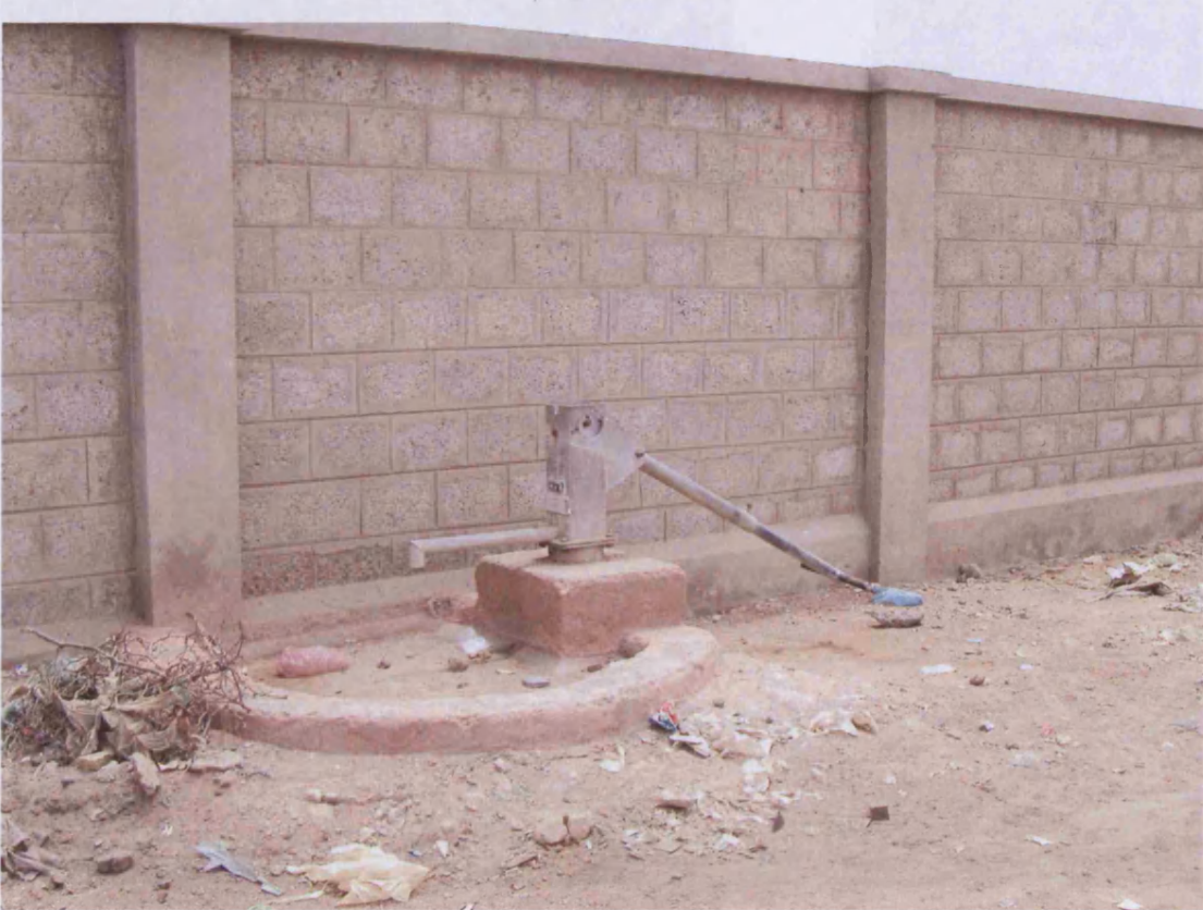
Figure 2.5 Infrastructure development as settlement consolidates.
