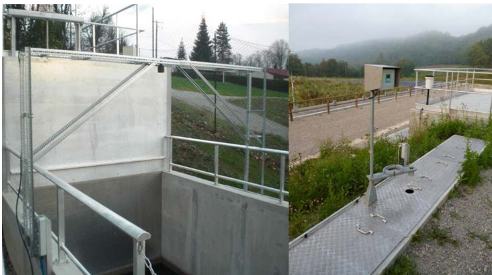
Figure 43: Flowmeters on the rainfall event system (left) and dry weather system (right)
