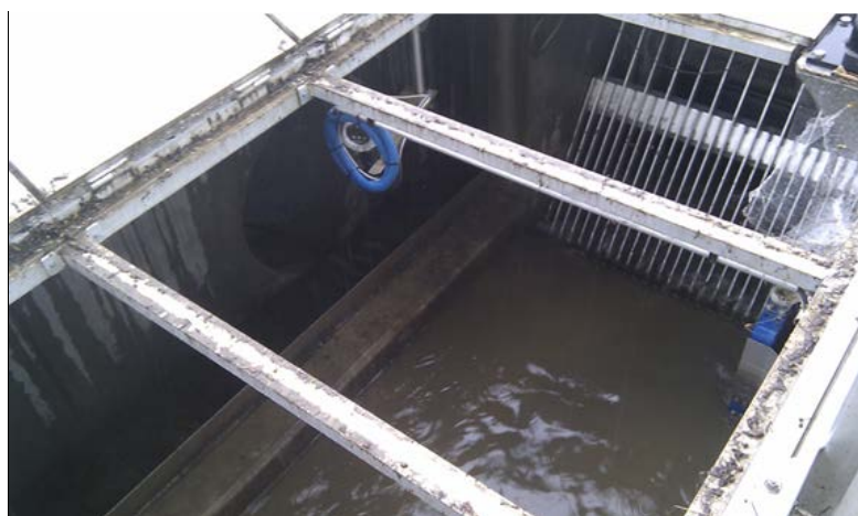
Figure 39: CSO of Challex plant in a storm event
