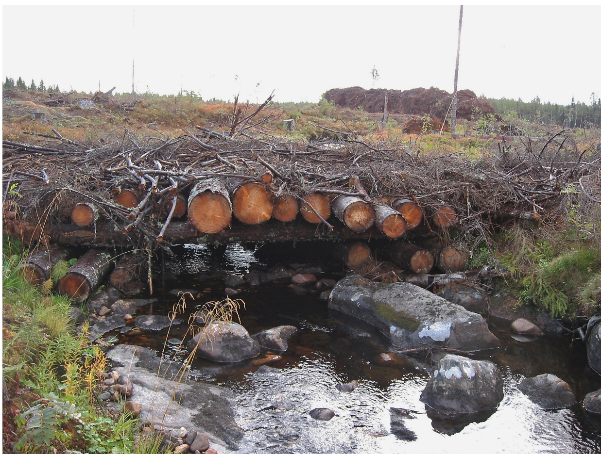
Figure 3. Temporary bridge. Photo: Börje Pettersson
