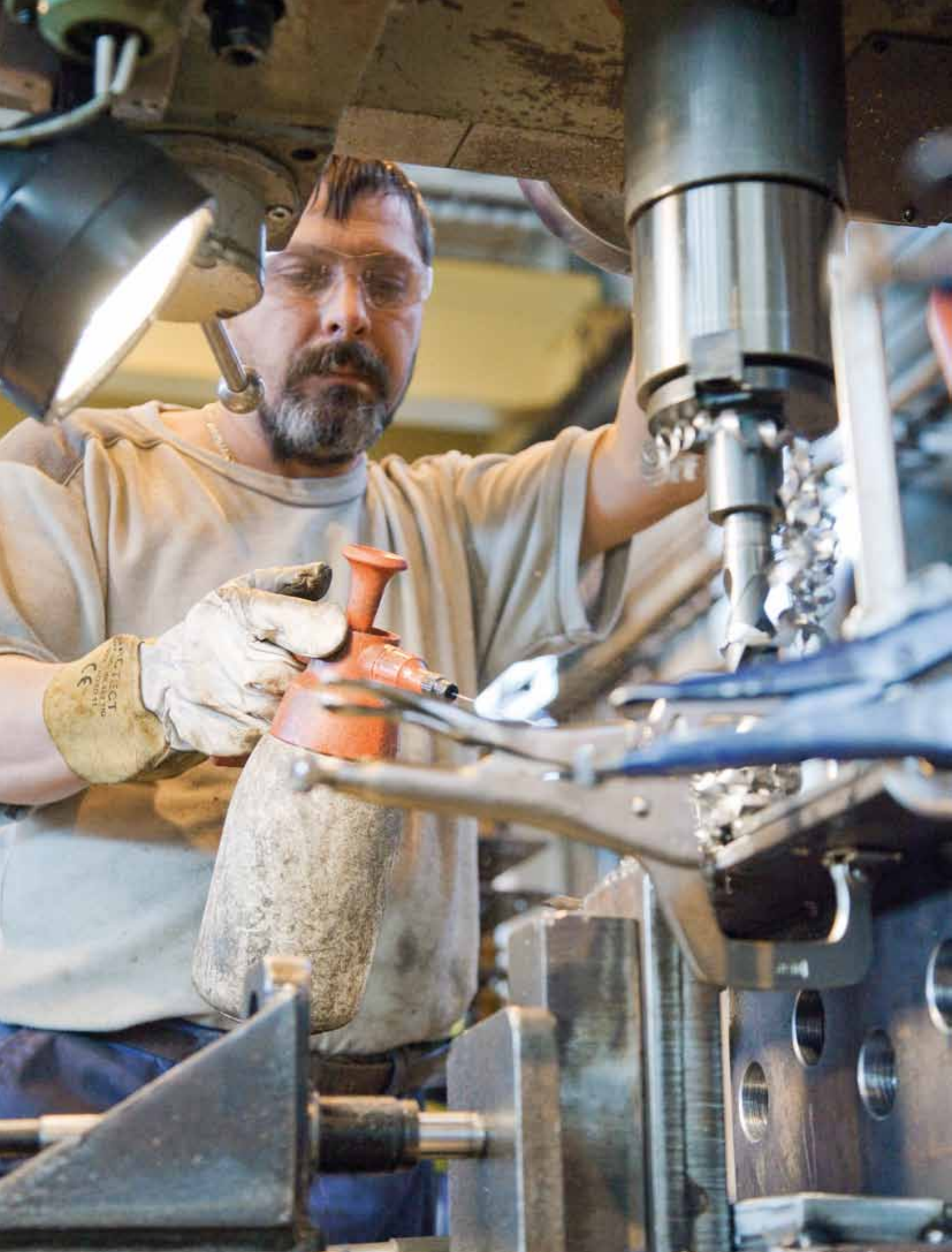
Foreign labour are also employed in the metal industry. Lázár Tibor drilling holes to a main girder at Miilupipe Oy in Raahé.
