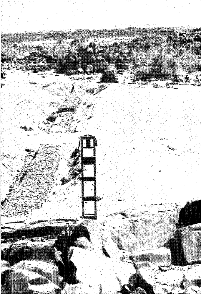
Figure 13.7 Reference station of the kori Teloua—carrying out a locking by 'gabions' (Air, Niger Republic)
