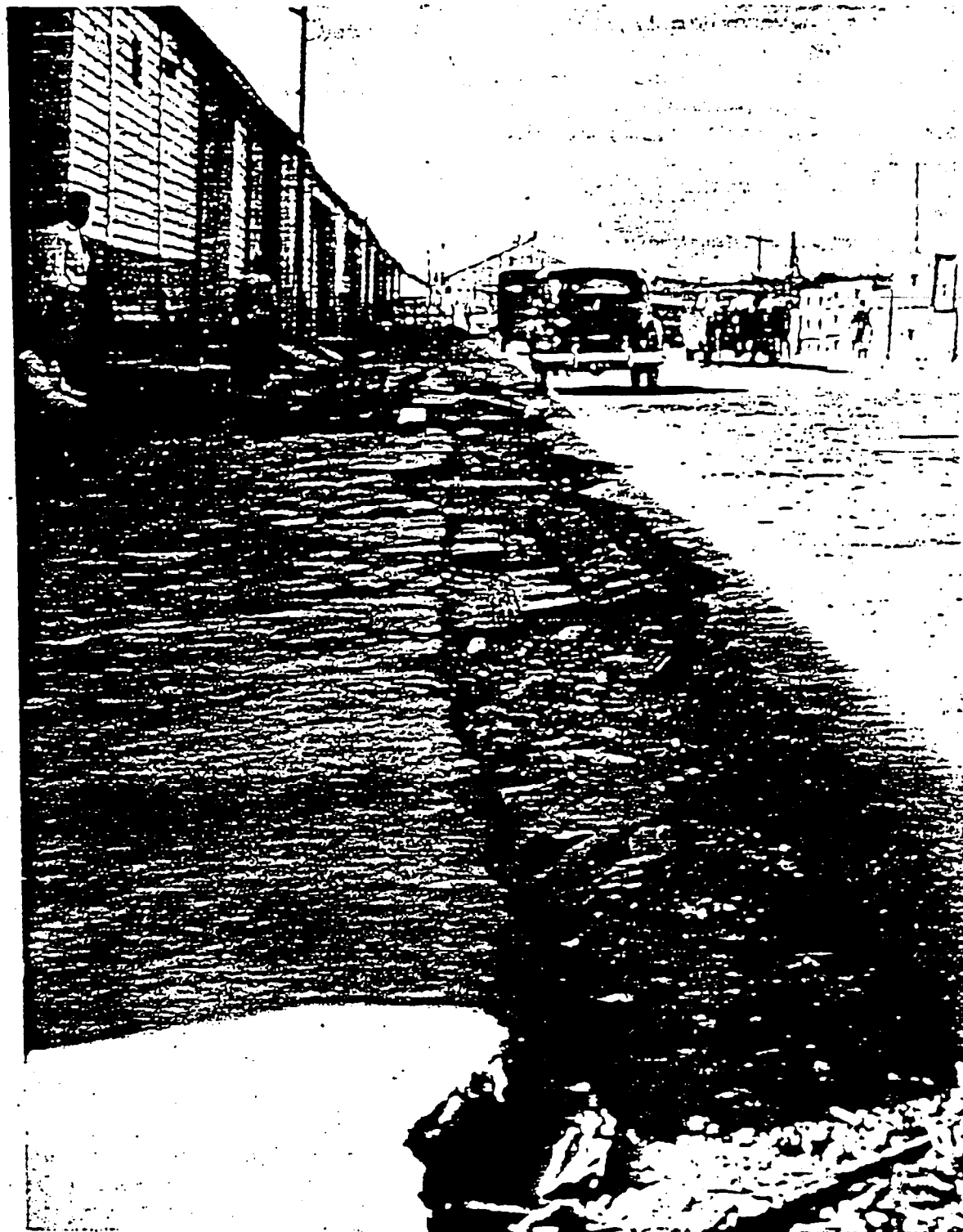
Damage at Suva wharf caused by the 1953 earthquake, which was followed by a tidal wave within 30 seconds.
