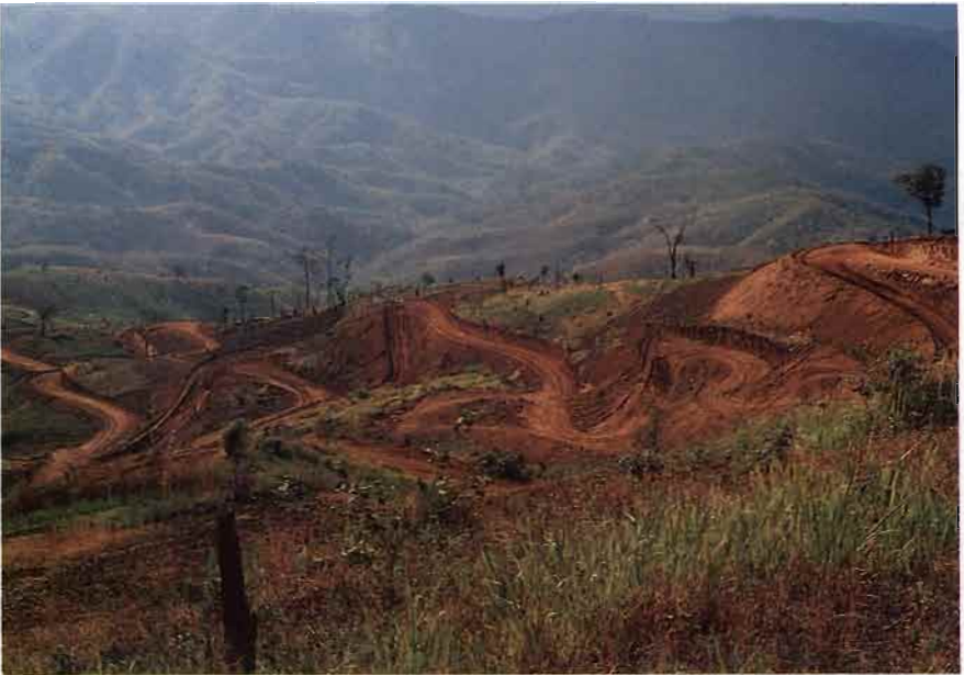
92. Road construction (McKinnon)
