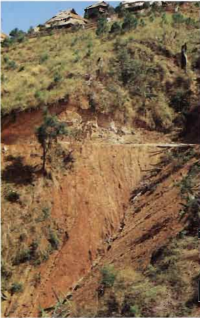
90. Road erosion, Doi Thung (McKinnon)
