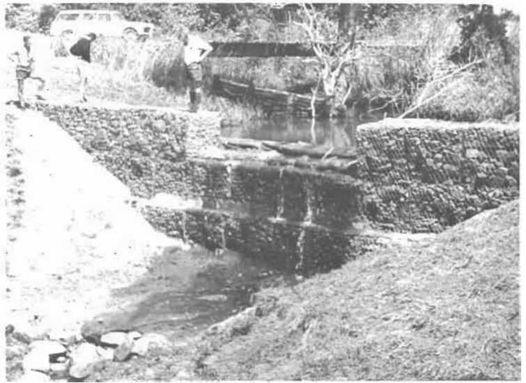
A gabion “drop structure” (right) stabilizing a streambed. The apron below the structure breaks the force of falling water. A good stone/grass lining (below) in a waterway can permit runoff to flow at high speeds without eroding the soil.
