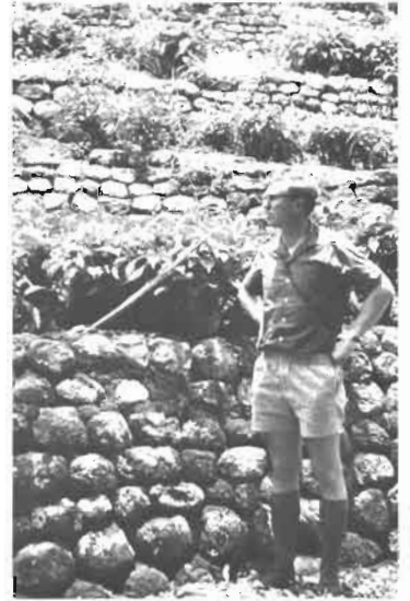
Bench terraces for tea protected by grass facing (left), and stone walling (above).
