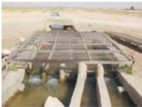
Structure to divide the qanat flow
