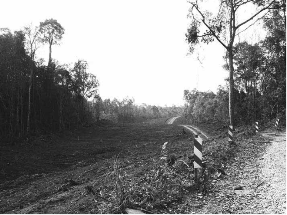
Figure 4.5 Excessive road clearance
