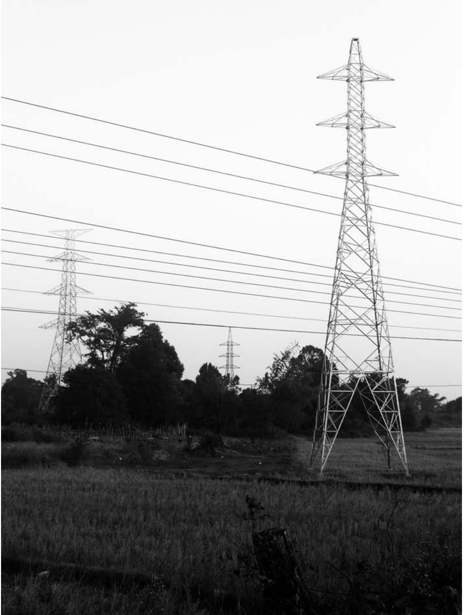
Figure 4.1 Nam Theun 2 Transmission tower
