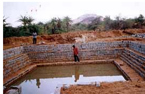
Tank at Kothagudikunta
