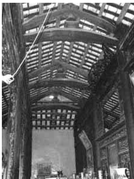
A frame of a traditional house with 8 wooden pillars at 18/9, Neighbourhood 7, Nha Be town
