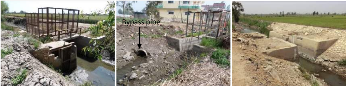
Figure 61. Hydraulic structures in disuse, bypassed, or removed in IIP areas.
