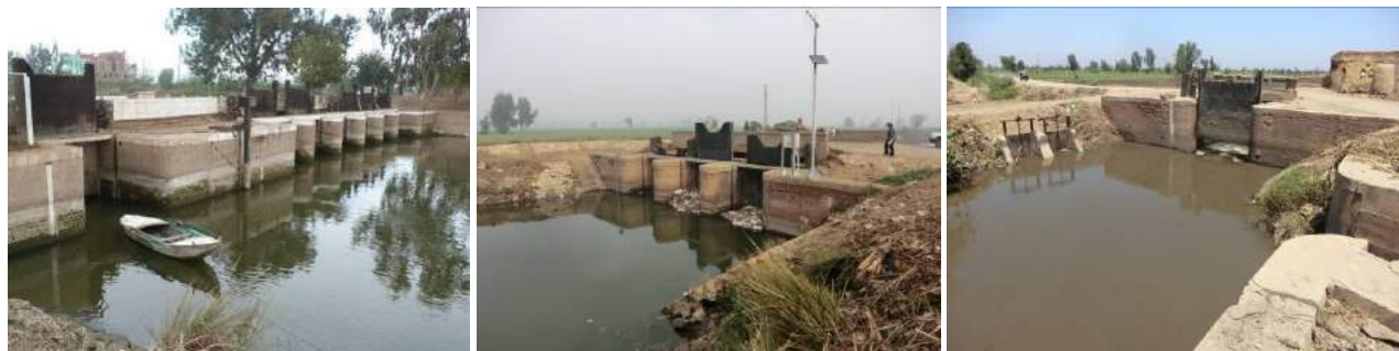
Figure 7. Snapshots of some main regulation structures (Beltag, on Zawiya, on Bosees)
