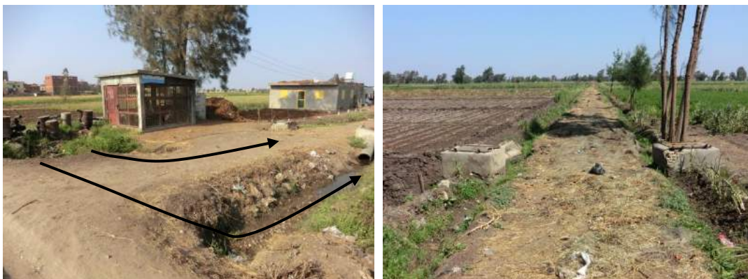
Figure 12. Valves and distribution pipes along the branch canals
