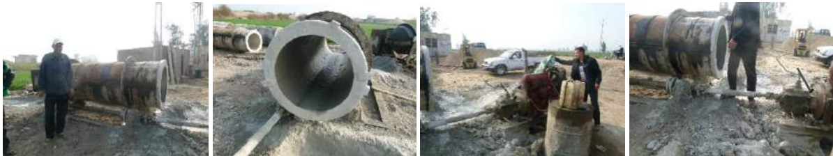
Figure 14. Local production of big pipes for mesqas
