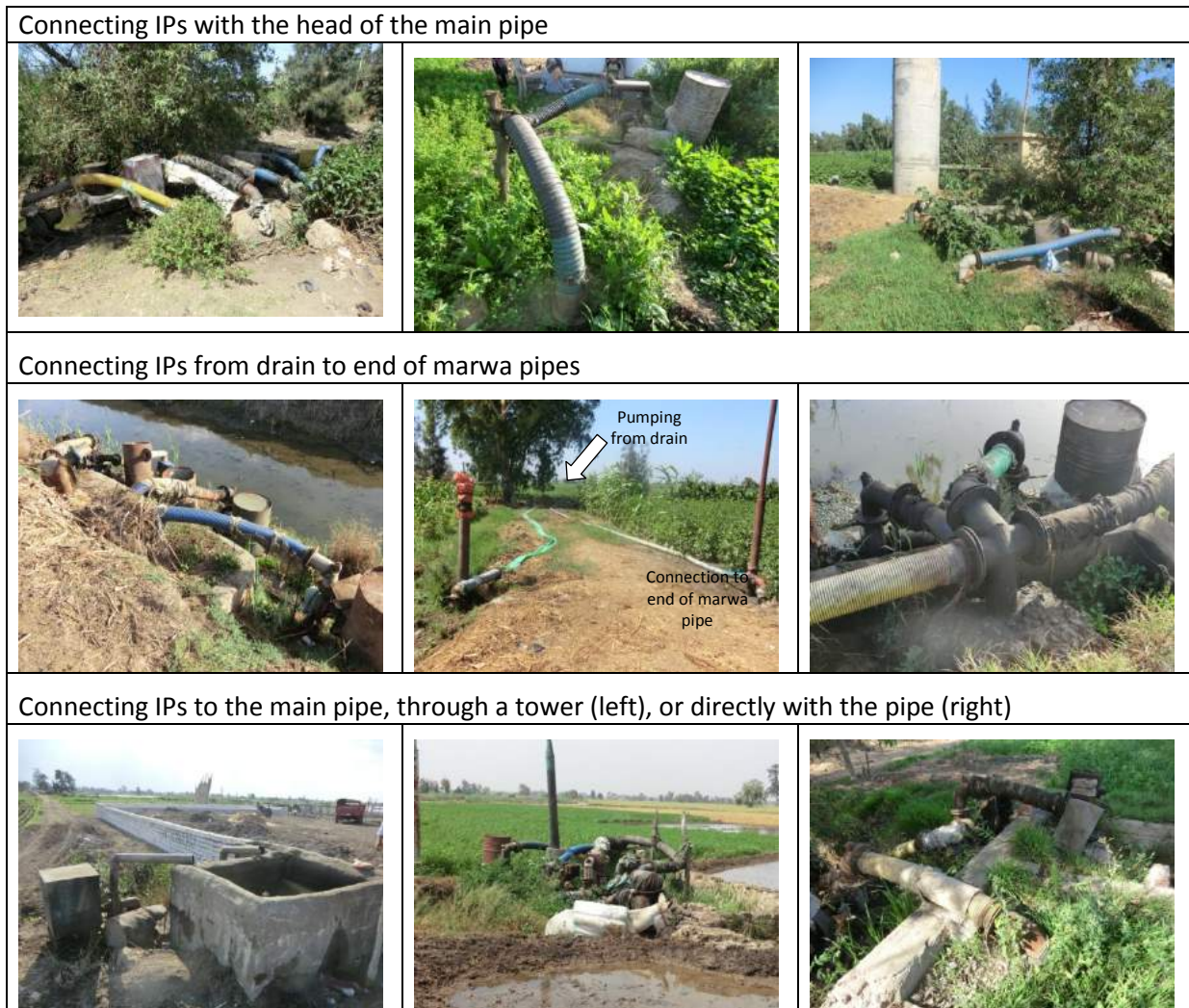
Figure 20. Connection of IPs to the distribution network
