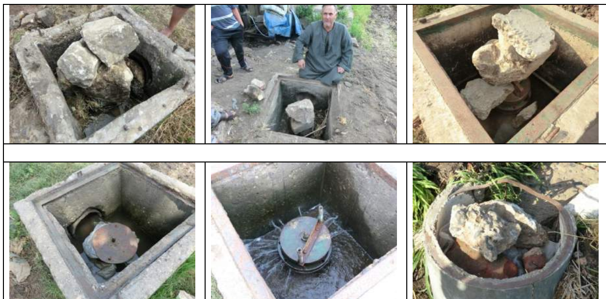
Figure 29. Problems of leakage with alfalfa valves
