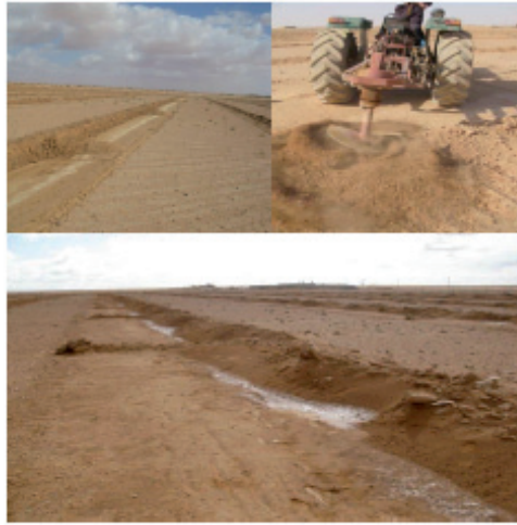
Figure 5. Site preparation for the project area
