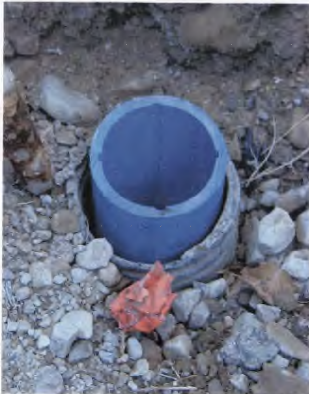
Fig. 3.31 Additional photographs showing the recovered inclinometer I2 casing
