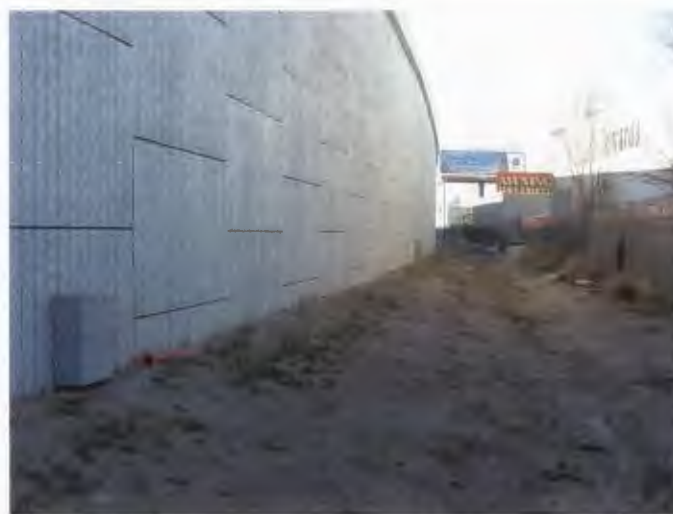
Fig. 1.3 Photographs showing Wall R-346-1C during and after construction
