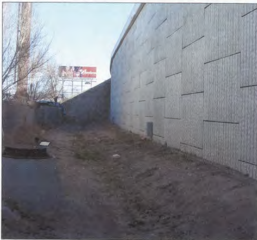
Fig. 3.19 Views from the north and south, respectively, showing the two electrical boxes containing strain gage cables and connectors for the two instrumented sections of wall
