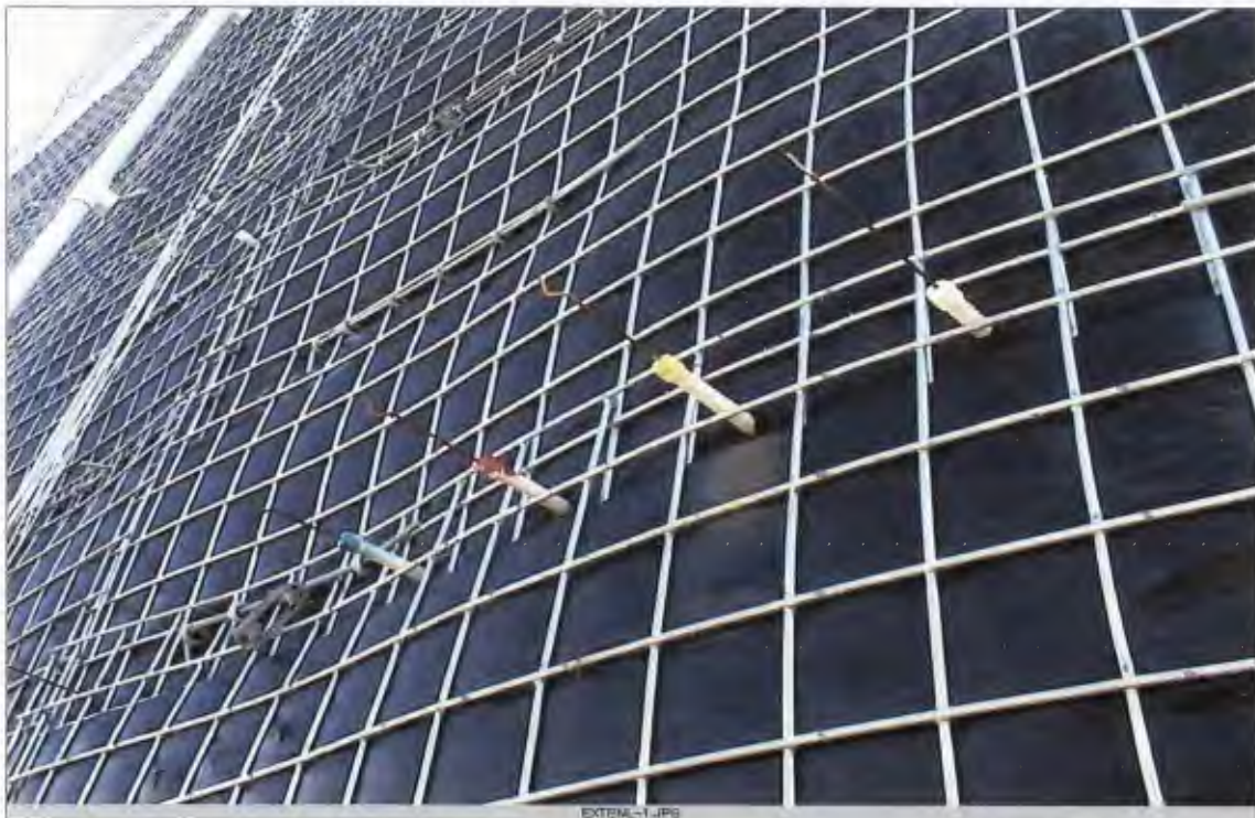
Fig. 3.13 Photograph showing horizontal extensometers protruding from wall face
