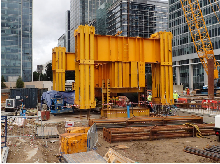
Fig. 2 Static load testing frame for the trial test pile (reproduced from de Battista et al. [29] with permission).
