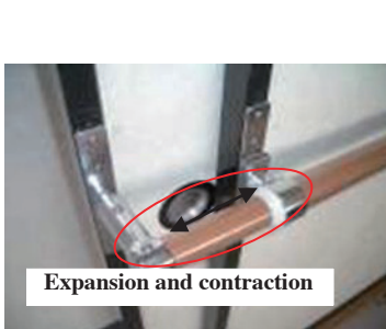
Fig. 3 Extendable handrail
