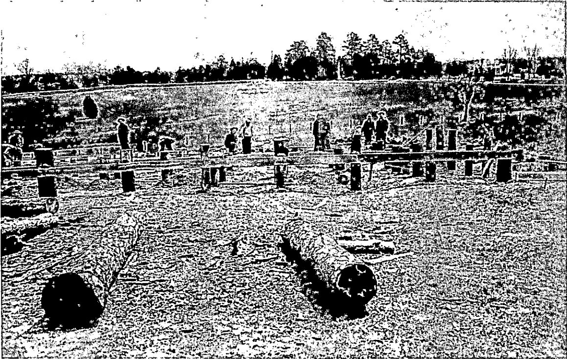
VIEW OF VIEWING AREA UNDER CONSTRUCTION PHOTOGRAPH CURTESY OF JULIA STEELE
