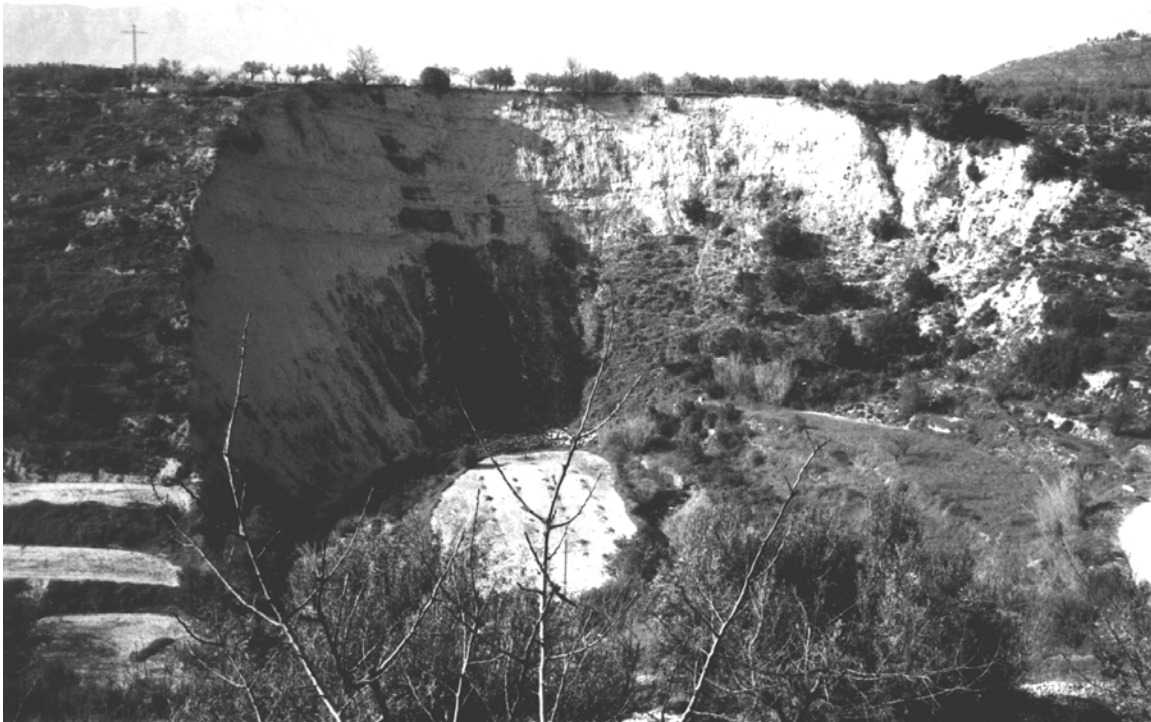
Plate 5: Undercutting and removal of material from an unstable slope
