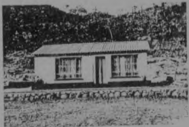
9b. kaNyamazane: Bigger windows have replaced the originals. Benches built against the walls either side of the front door.
