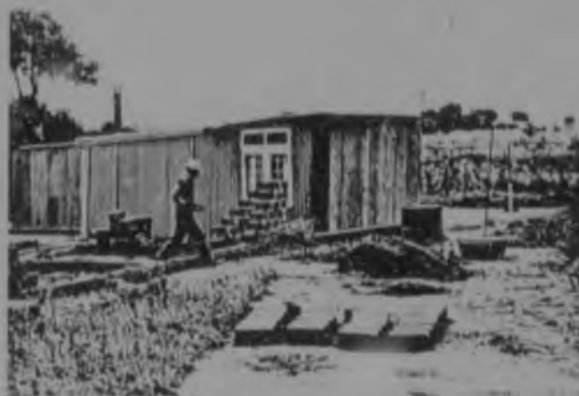
1b. Winterveldt: Temporary dwelling next to the foundations of the permanent house.
