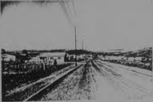
22a. Main bus-route through Ngangelizwe tarred and provided with stormwater drainage.
