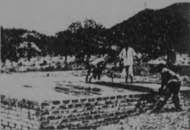
51f. Completing a plinth. Contractors train their own work teams.
