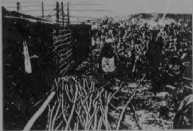
36d. A woman assisting a contractor with erecting a wattle framework
