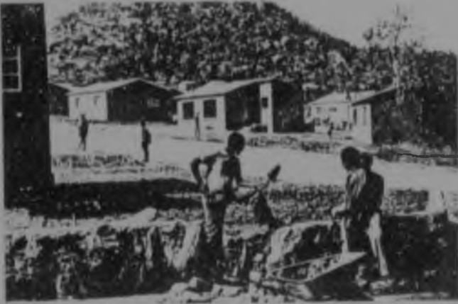
59a. Building a garden wall.
