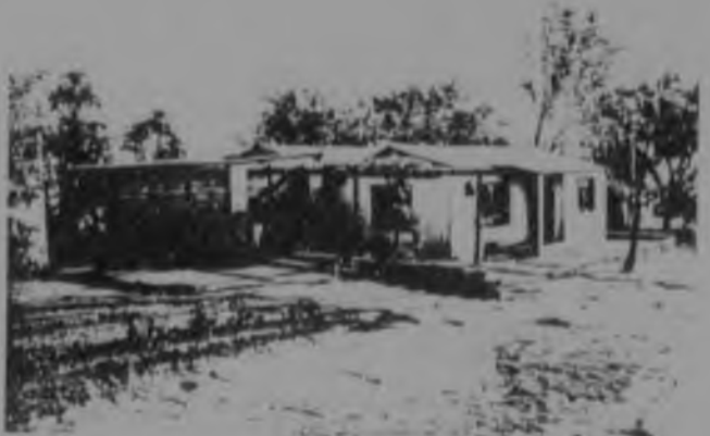
60d. Addition of extra accommodation in front and a garage on the side.
