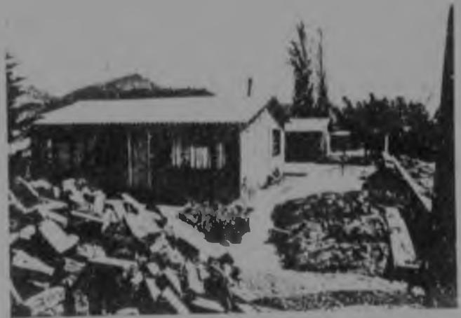
60g. Larger windows installed and materials stockpiled for additions, 1978.
