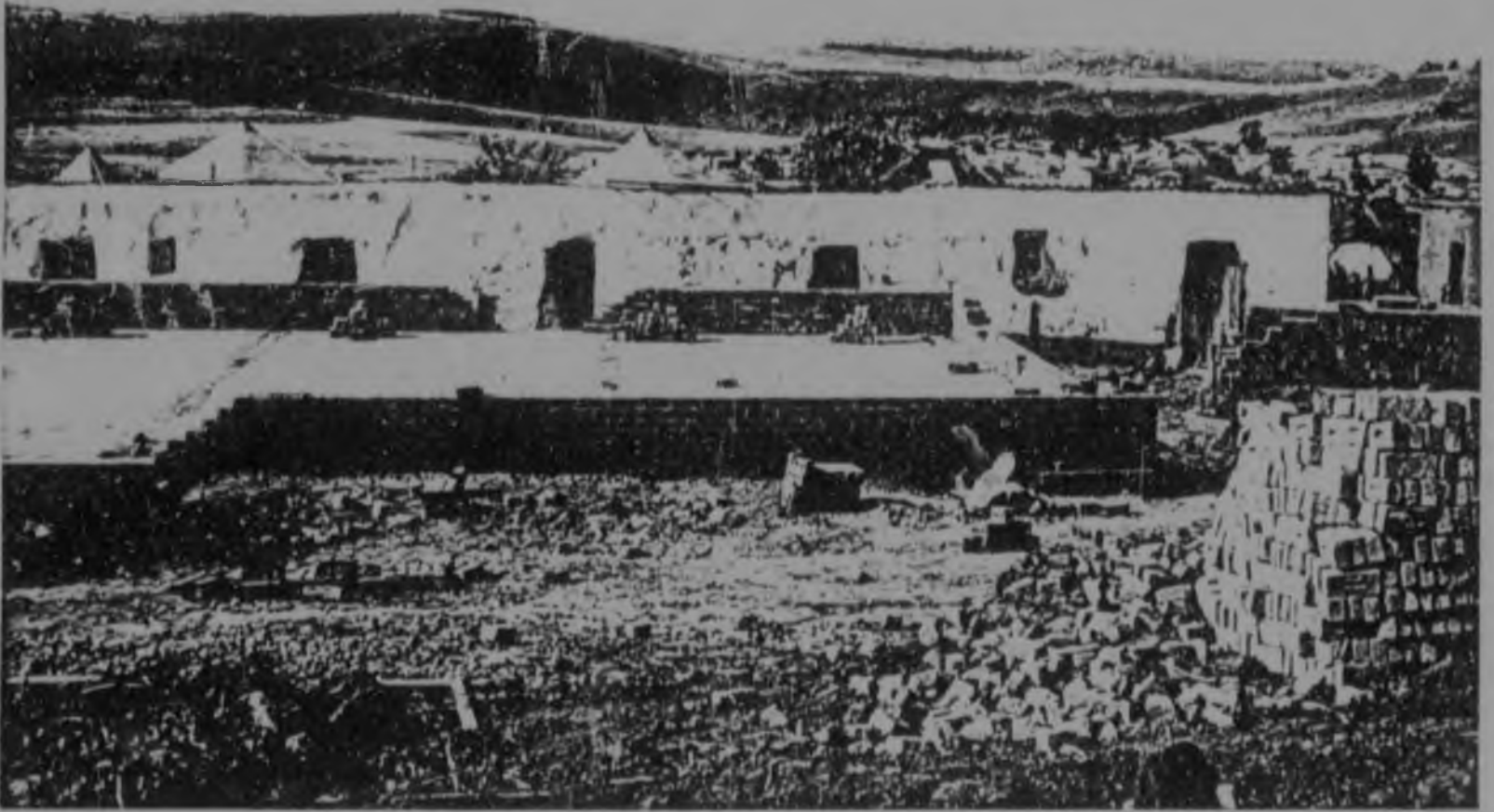
38a. Row of wattle and daub 'flats' which are let out to provide an income. One is occupied by the site 'owner'. He is in the process of erecting a large 'modern' home in the front of the site
