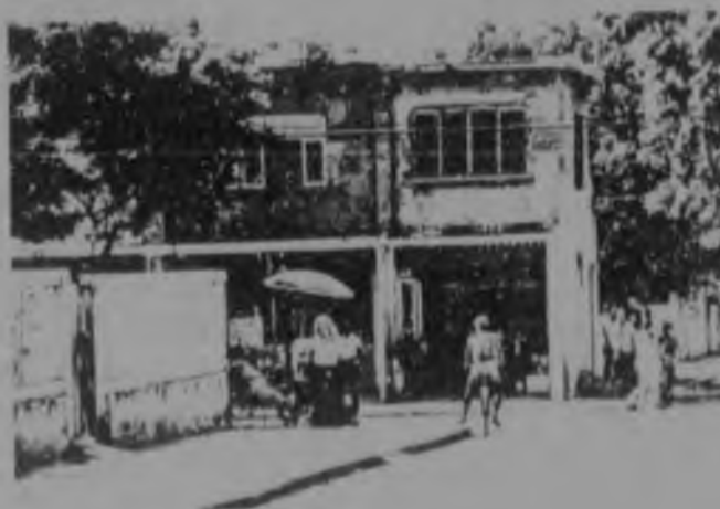
11d. Vila Kennedy, Brazil: Houses built on an upper level. Space below used for expanding accommodation or economic activity.
