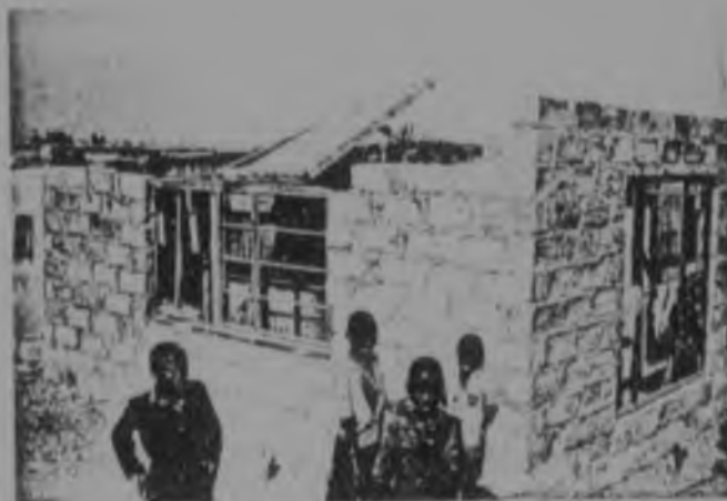
1h. Winterveldt: Walls of the permanent house being erected around the temporary one which will later be removed. (NBRI)
