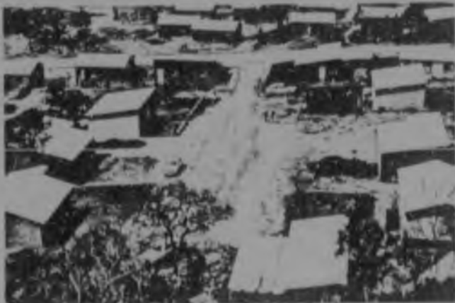
55c. Forecourt shared by ten employees of one company shortly after occupation, May 1978.
