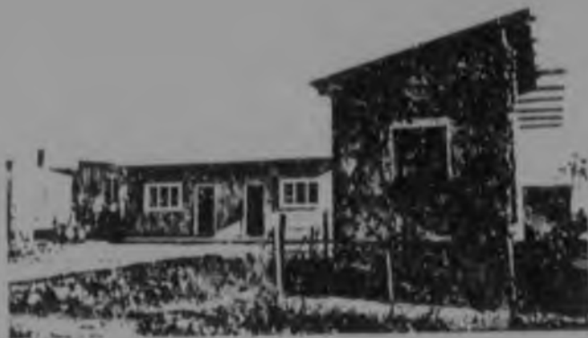
38d. Site on left is 'flats' at the back. Site on the right is an owner-built core-house.
