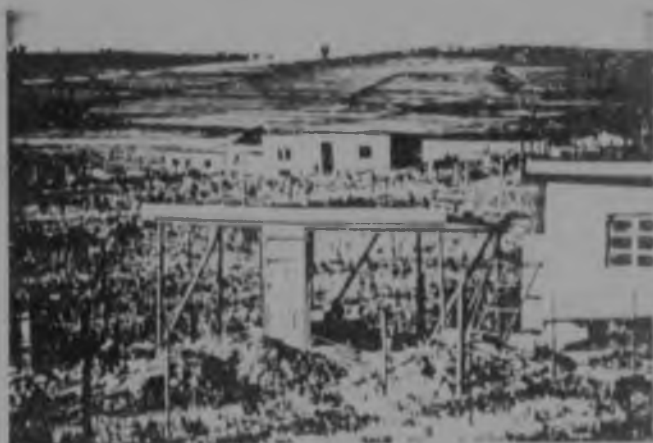
1d. Rural Transkei: Roof on supports completed To be filled in later.
