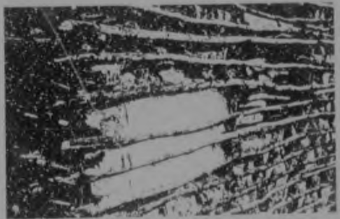
36c. Cement-based plaster improves the performance of a wattle and daub structure. (NDRR)
