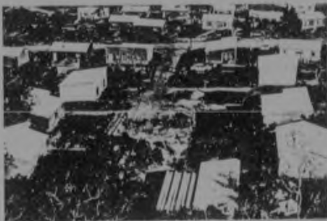
55e. Same forecourt in September 1979. Stones have been delivered for improving the edges and lining of stormwater channels.
