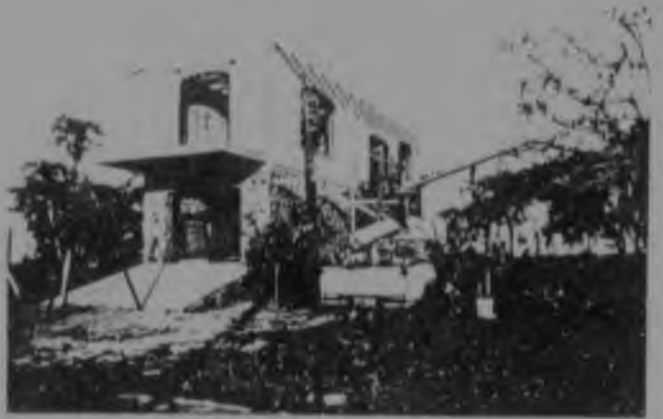
60c. A garage with extra accommodation above. Built behind a standard 51/9 type.
