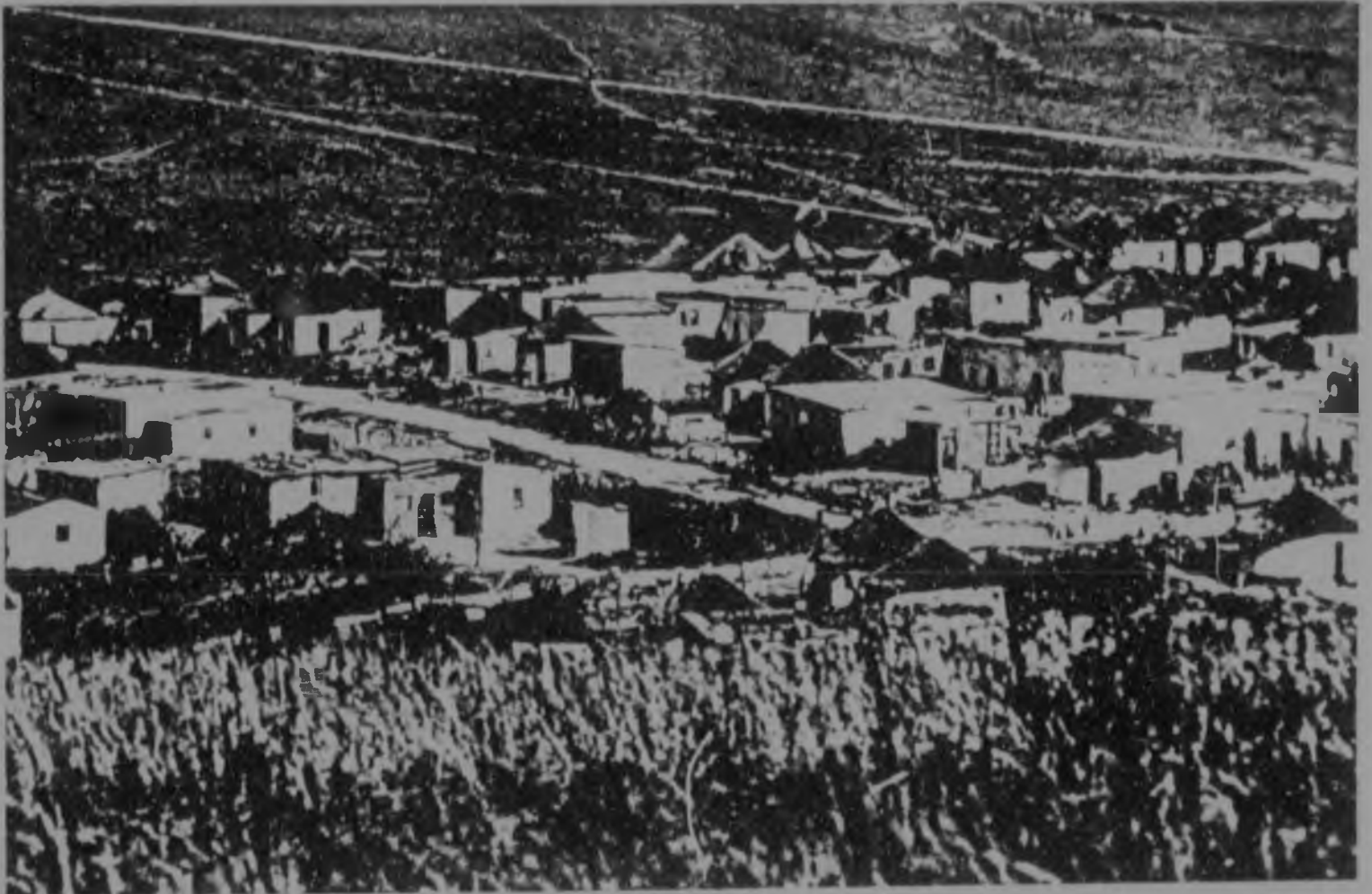
21c. Ngangelizwe: Note the range of built form. Mixtures of traditional and Western building-types and technology. (NBRI)
