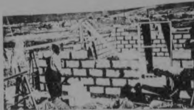
36f. Conventional brick construction.
