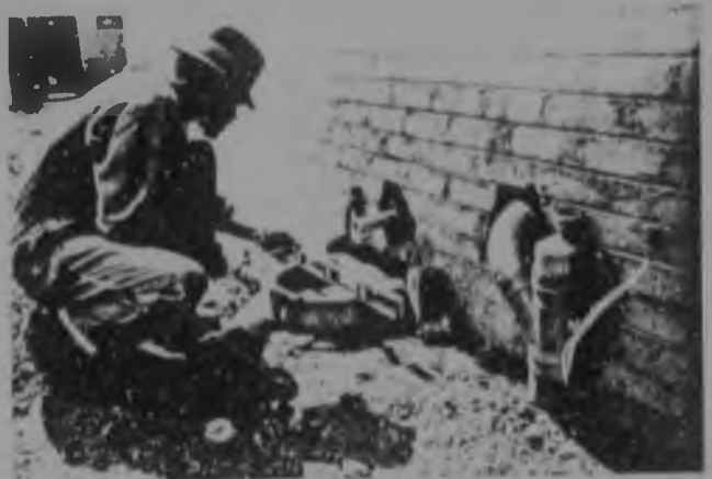
51j. Plumbing contractor
