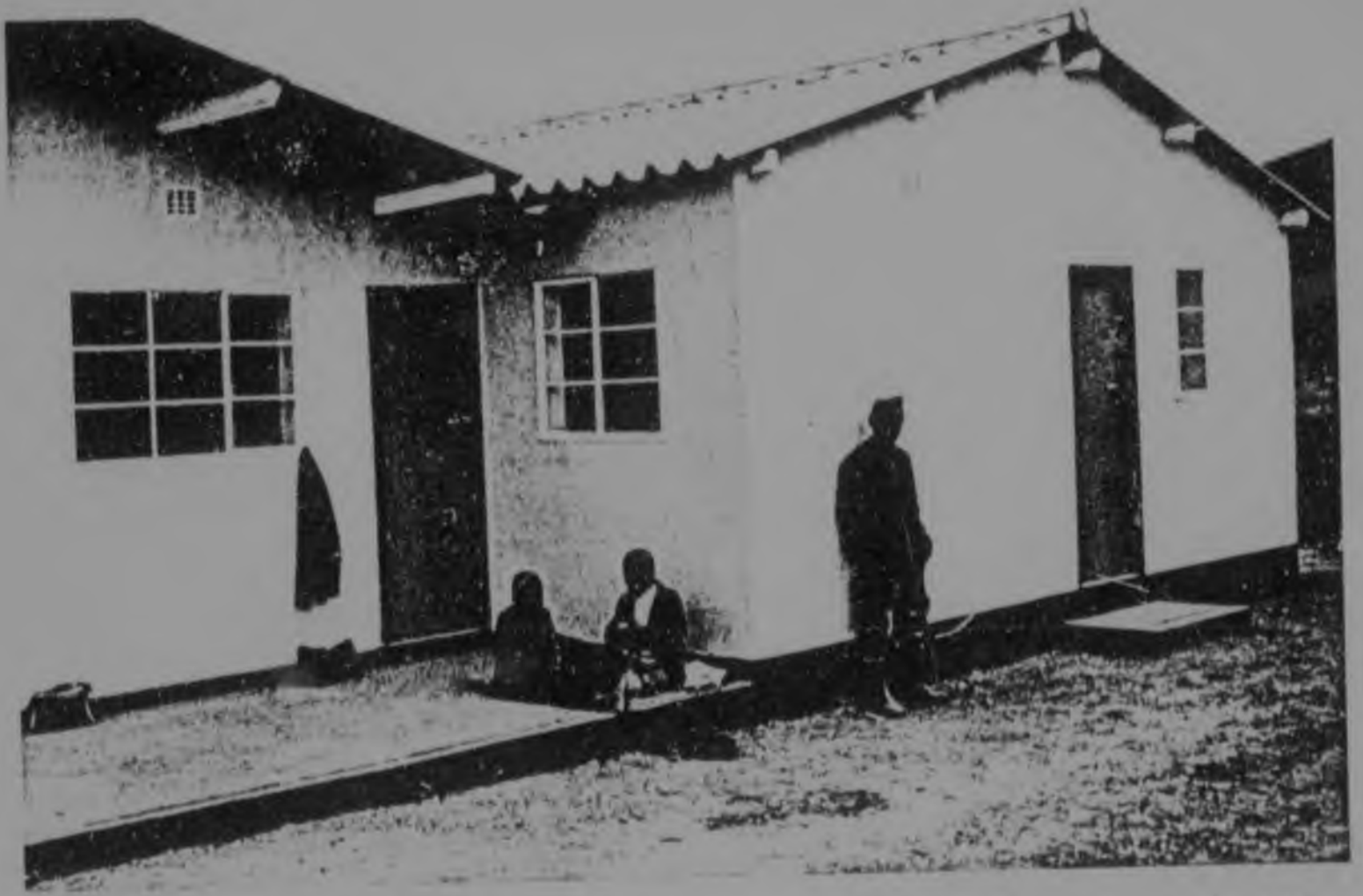
Ada. Demonstration of an addition to a standard 31/9 house-type with the use of a single sheet of 'Canalic' as a box-gutter.
