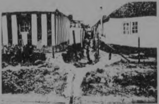
24. Water stand-pipe to each house Service lane between houses for night-soil removal.
