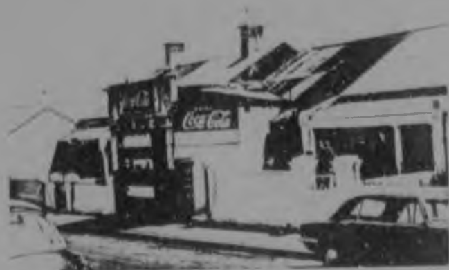
11b. Observatory, Cape: Small shop built onto a house.
