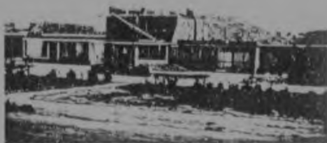
1e. Lima, Peru: Ground floor of houses completed in stages. Upper floors then added.
