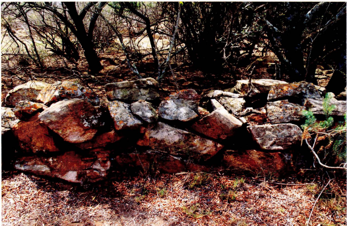
Figure 19: Low-walling of KD 21 inundated with soil and vegetation (shown in background).
