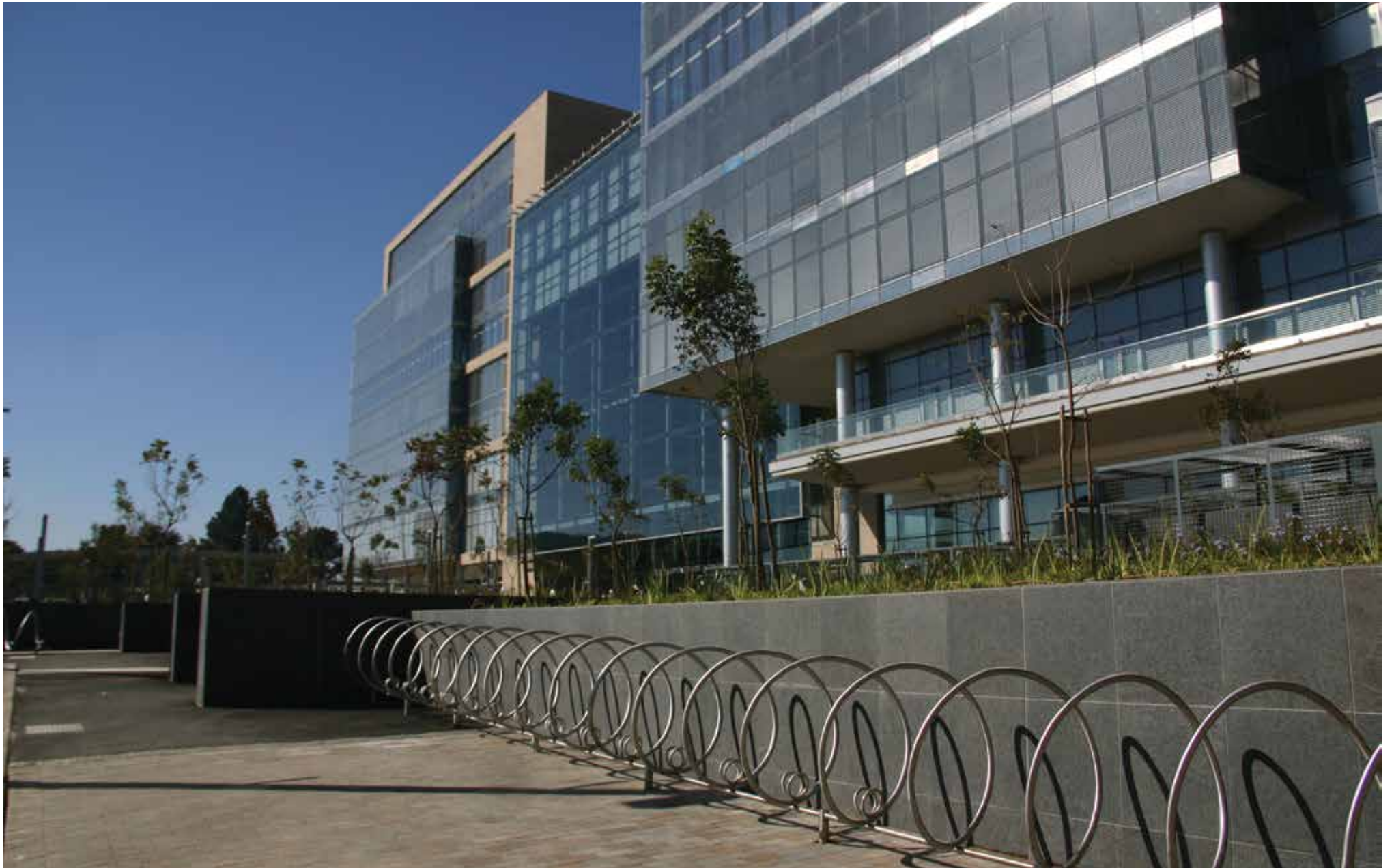
Figure 5.9: Bicycle racks at a newly constructed Standard Bank Building, Rosebank (photo taken before employees moved into the building). (Source: Christina Culwick)
