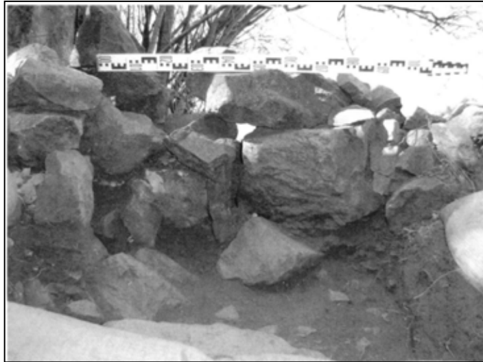
Fig. 4.6 Retaining wall excavation unit J-6, facing toward Vaal River (image Bradfield and Sadr 2011)
